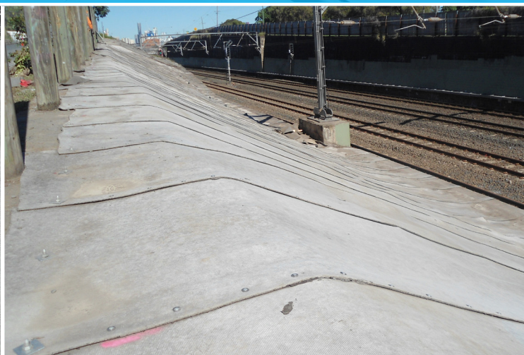
Screws and Sikaflex Pro were used to fix adjacent layers of CC
