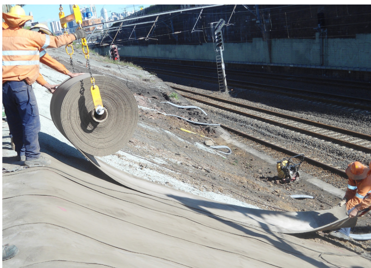
CC was unrolled and placed before being cut to length
