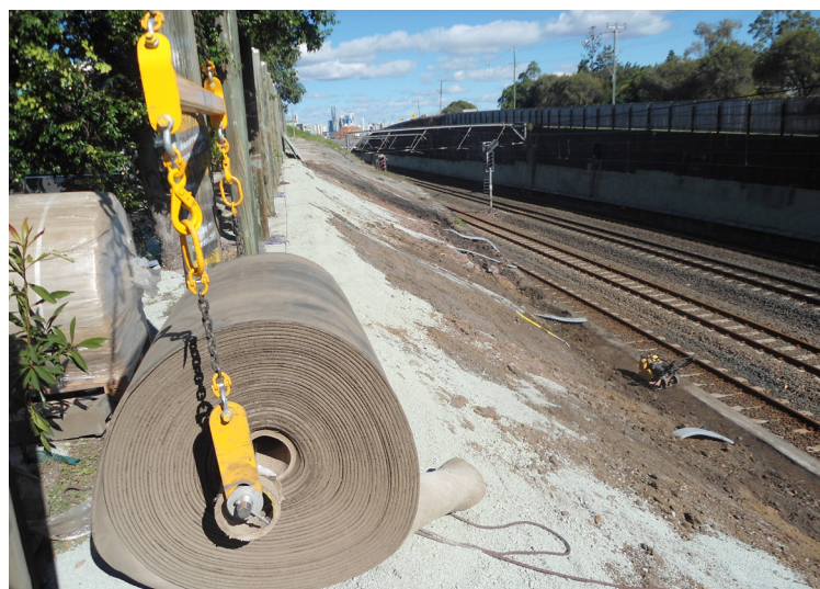
CC delivered on site in bulk rolls using a spreader beam and crane
