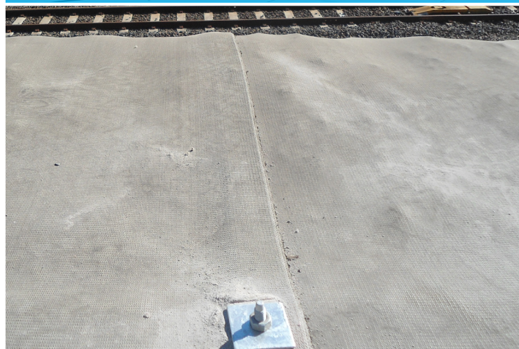
CC fixed at crest of slope with ground peg and washer
