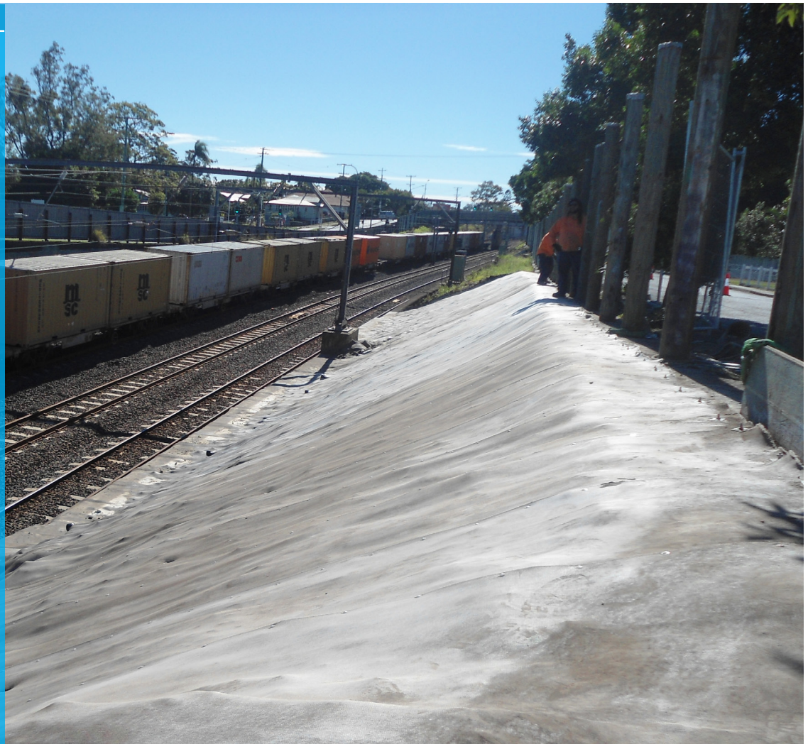
Completed section of slope lined with CC5
