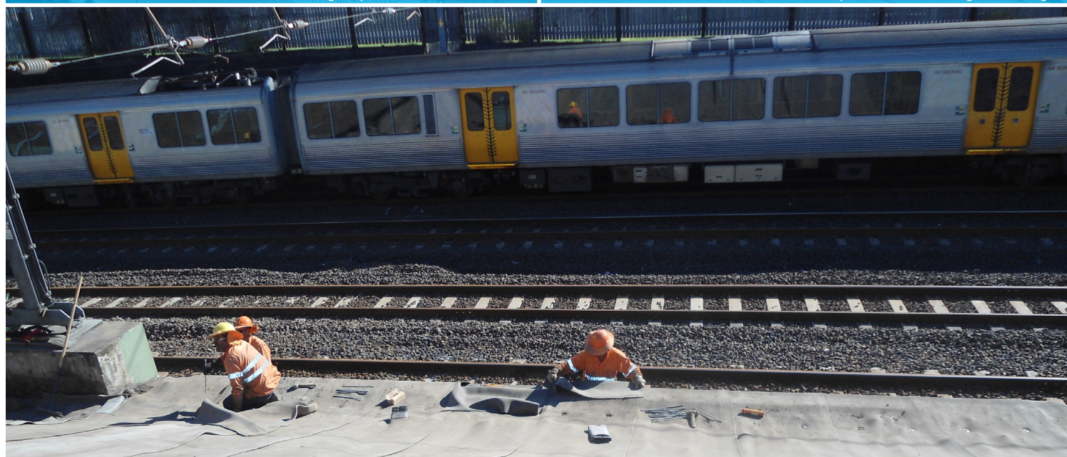
Using CC as an alternative to shotcrete enabled work to be completed without the need for a lengthy line possession
