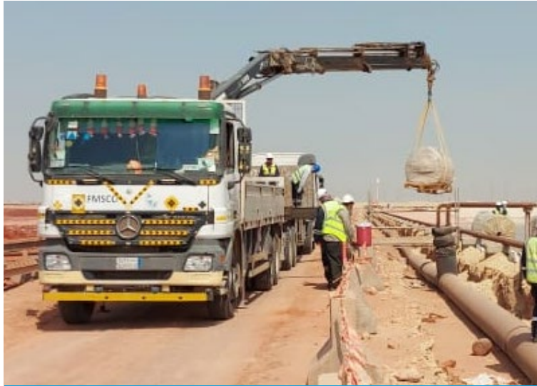
CC5™ Deployed using boom truck
