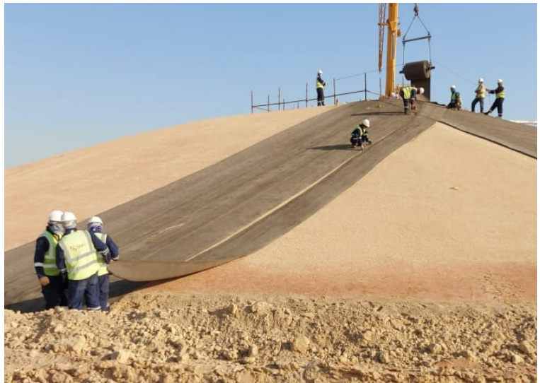
CC5™ Material laid vertically down the slope
