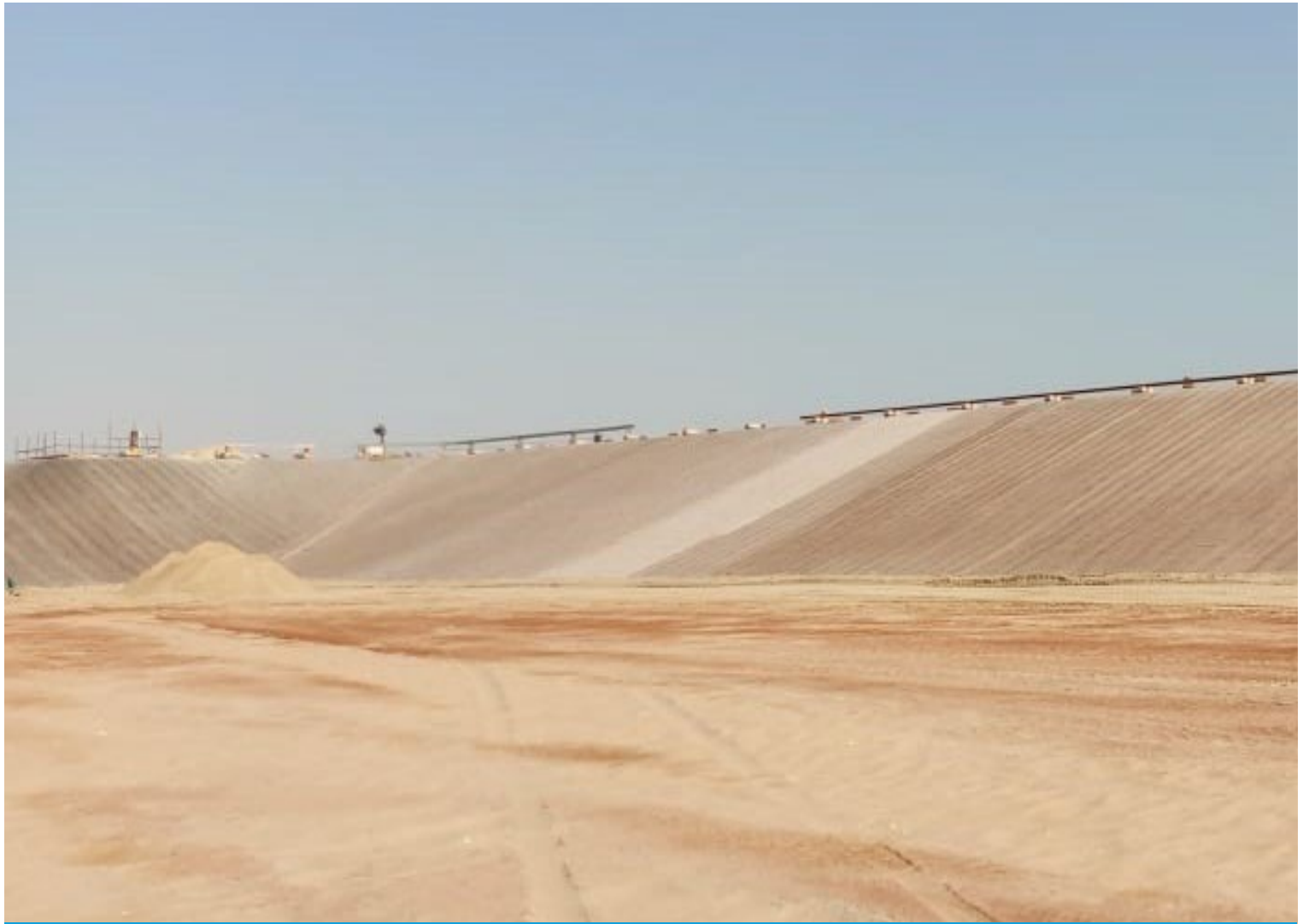
Completed slope protection works
