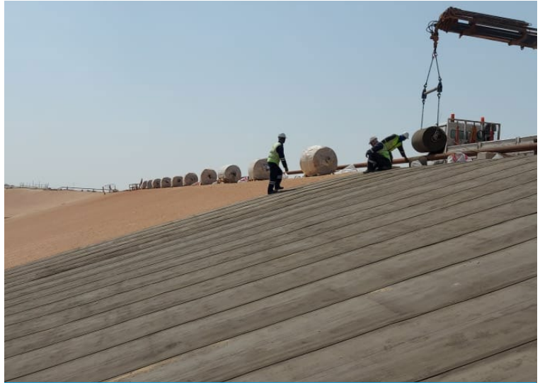
CC5™ Material suspended using spreader beam
