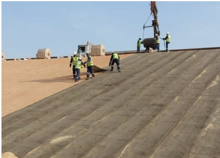
CC5™ Material laid vertically down the slope
