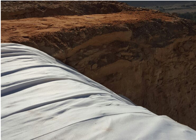
A geotextile was laid prior to installation of the CC
