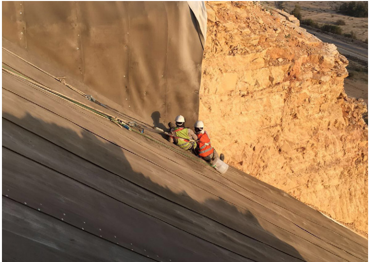
Contractors fixing the CC with bolts & pegs to the slope at 50mm centers
