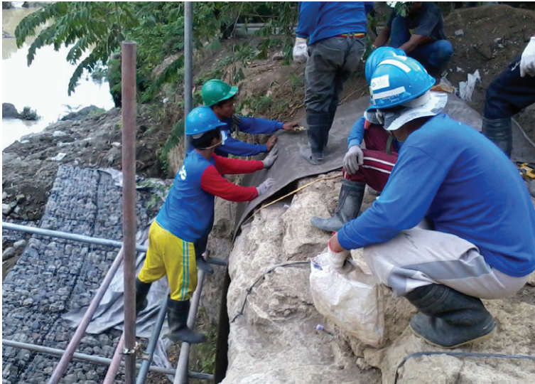
The CC was pegged into the anchor trenches
