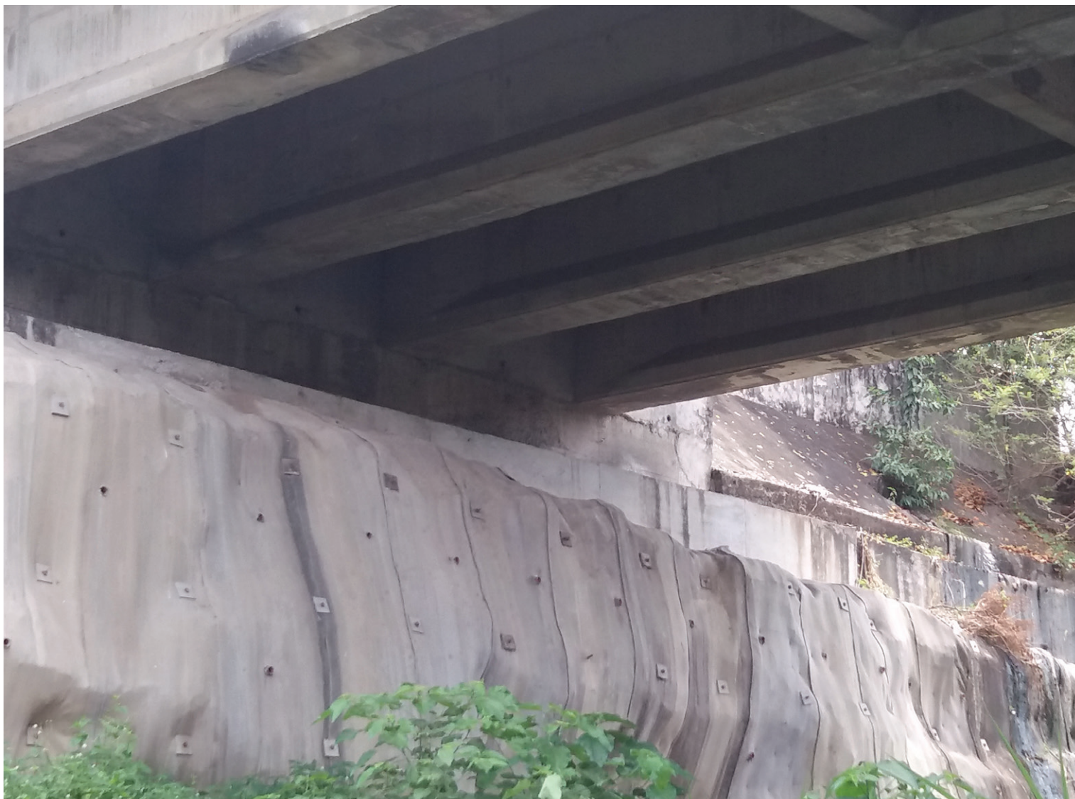
The complete installation, a further proposal including the use of CC was required for the other side of the bridge
