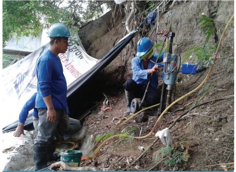
Holes were pre-drilled for the grouted anchors
