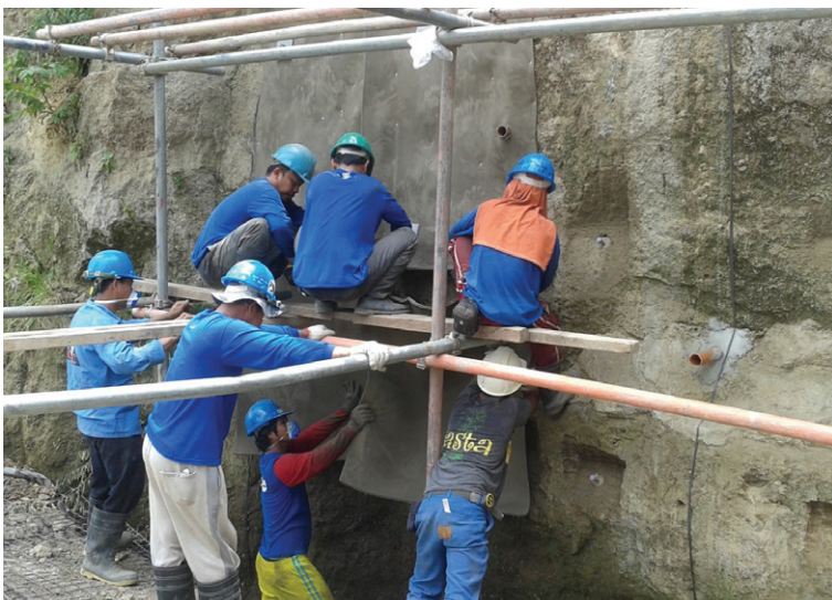
The CC was installed around the anchor protrusions
