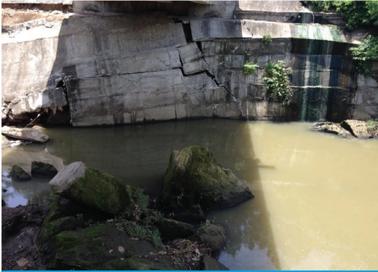
Existing damaged concrete lining
