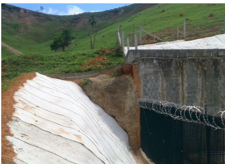
CC was installed on two sections of slope
