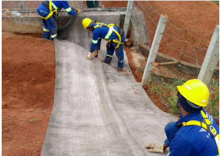
The CC was laid vertically down the slope
