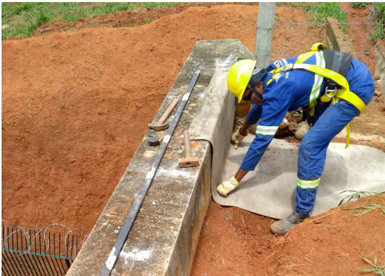
The material was laid flush to the substrate to avoid voids
