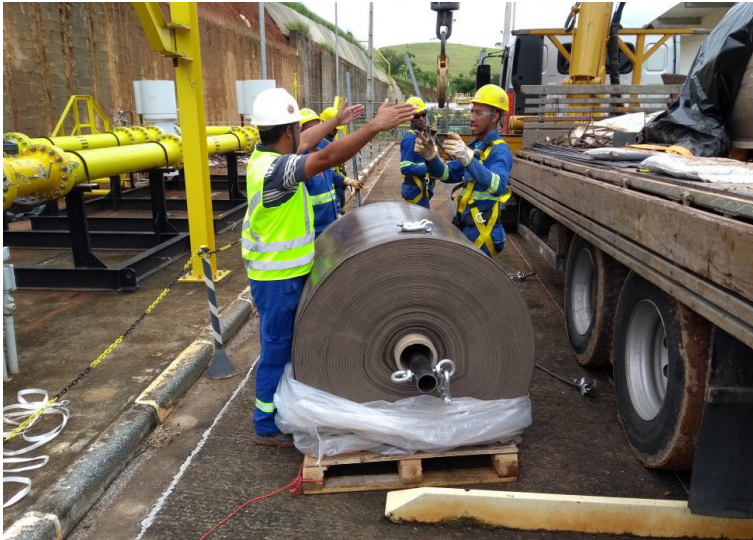
The CC was delivered in bulk rolls and mounted onto a spreader beam
