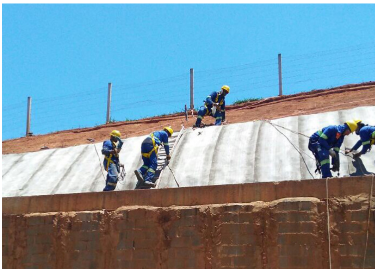
Climbing equipment was used to install the CC on the steep slopes
