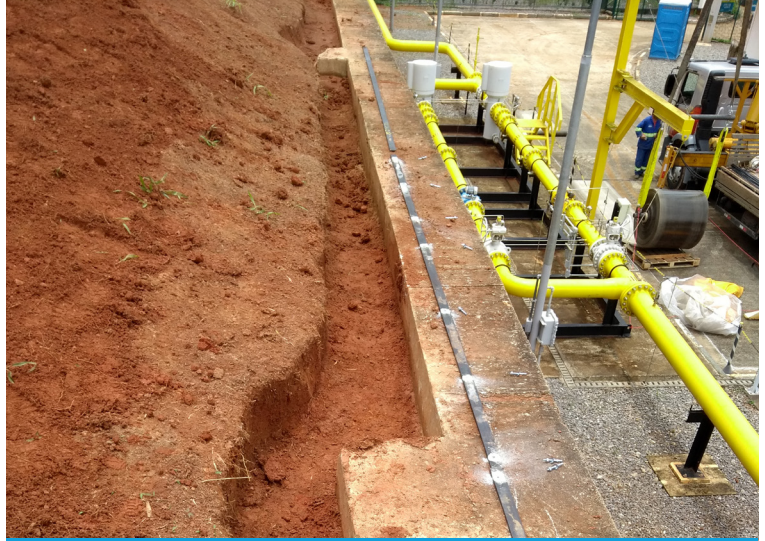
The pre-dug anchor trench
