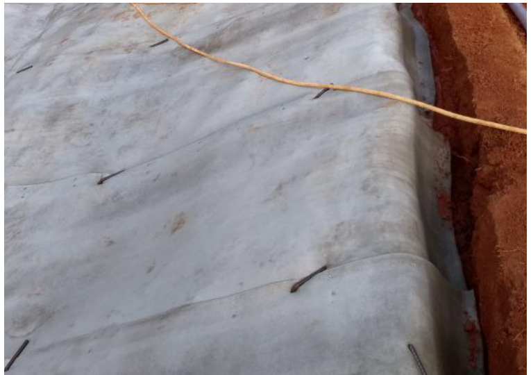
Ground pegs fixed the CC to the substrate
