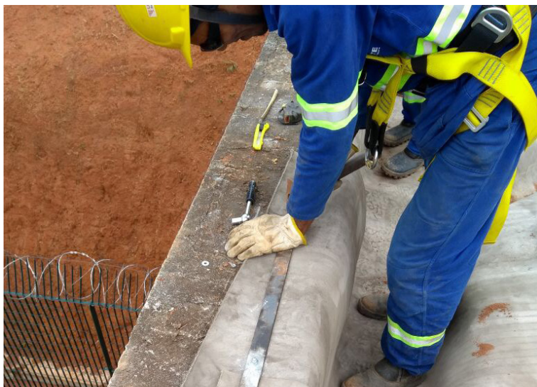
Anchor bolts were used to fix the CC to the wall at the toe
