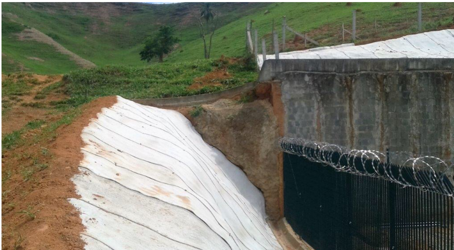
The two sections of completed CC-protected slope
