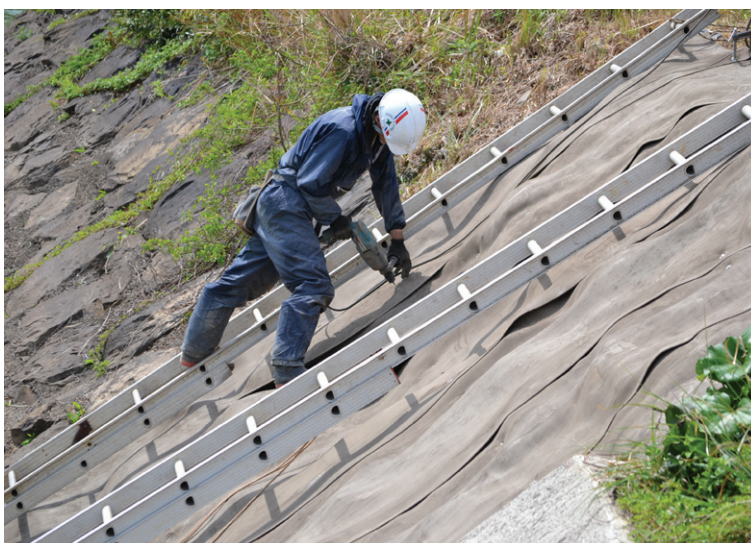
The CC was drilled, before being fixed with anchor bolts to the partial rock surface
