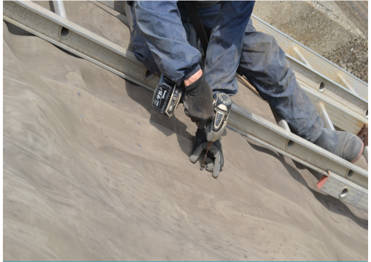
Screws were inserted at 200mm centers
