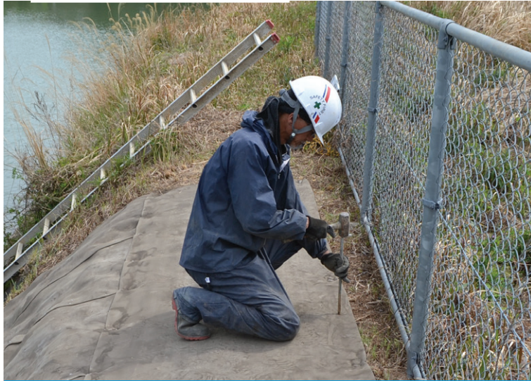
The CC was fixed at the top with steel anchor pegs
