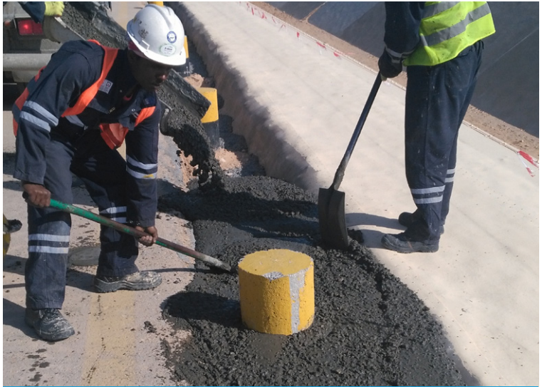
Anchor trench backfilled with concrete
