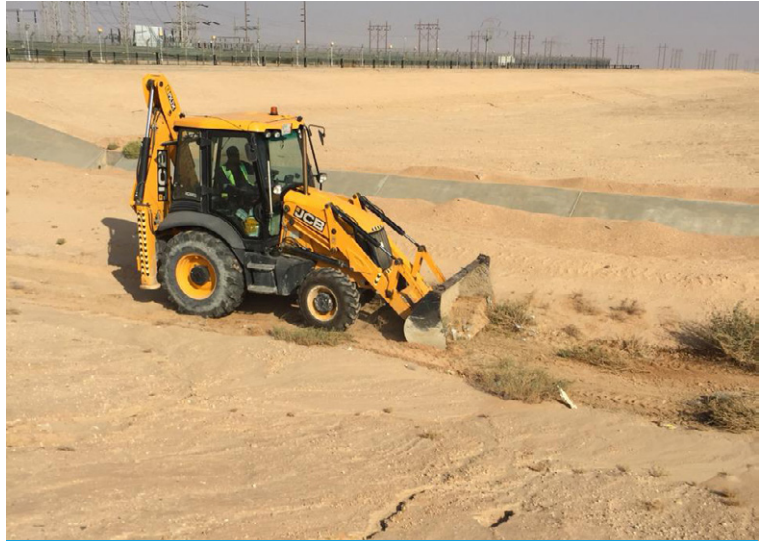
Vegetation removed using backhoe
