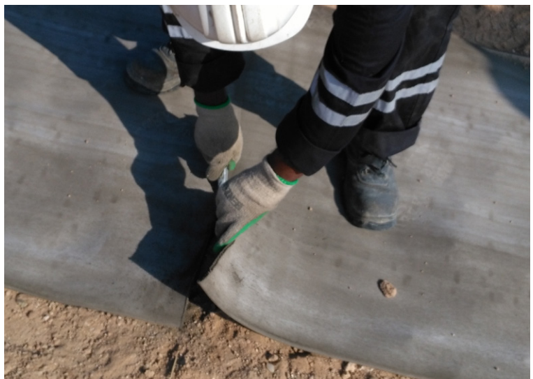
CC cut to length on site
