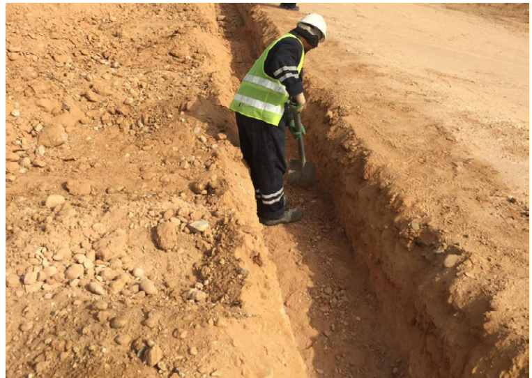
Anchor trenches dug by hand
