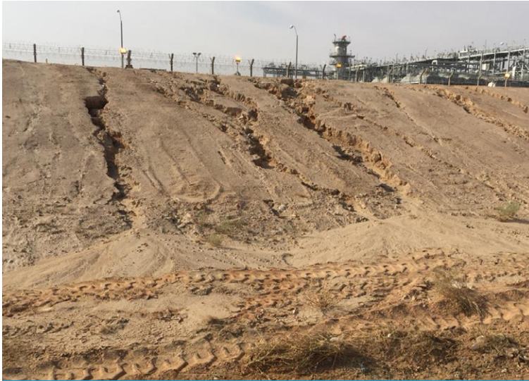
Slope had suffered weathering erosion
