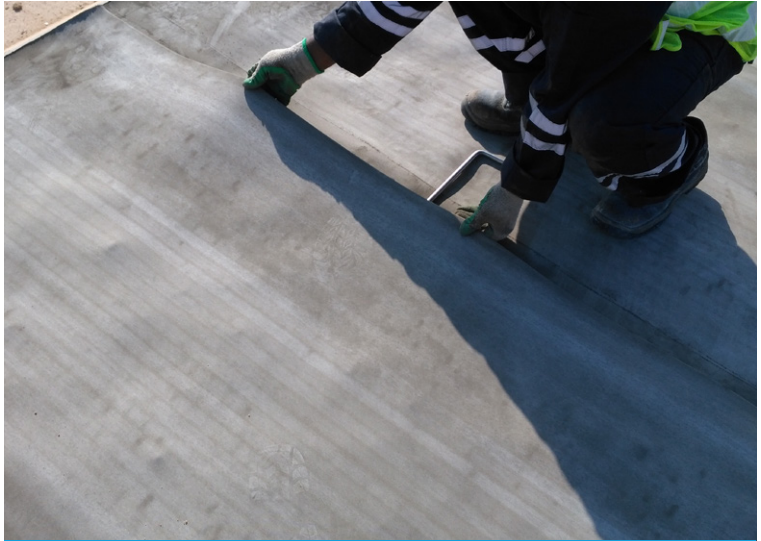
Subsequent layers overlapped by 100mm
