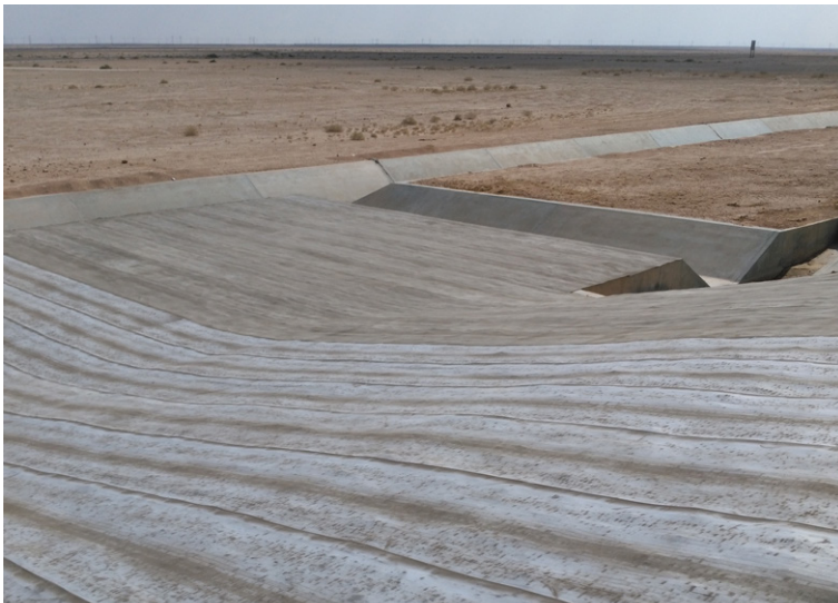
Section of slope following CC deployment
