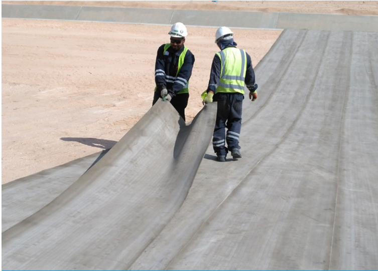
Batched CC moved into place by hand
