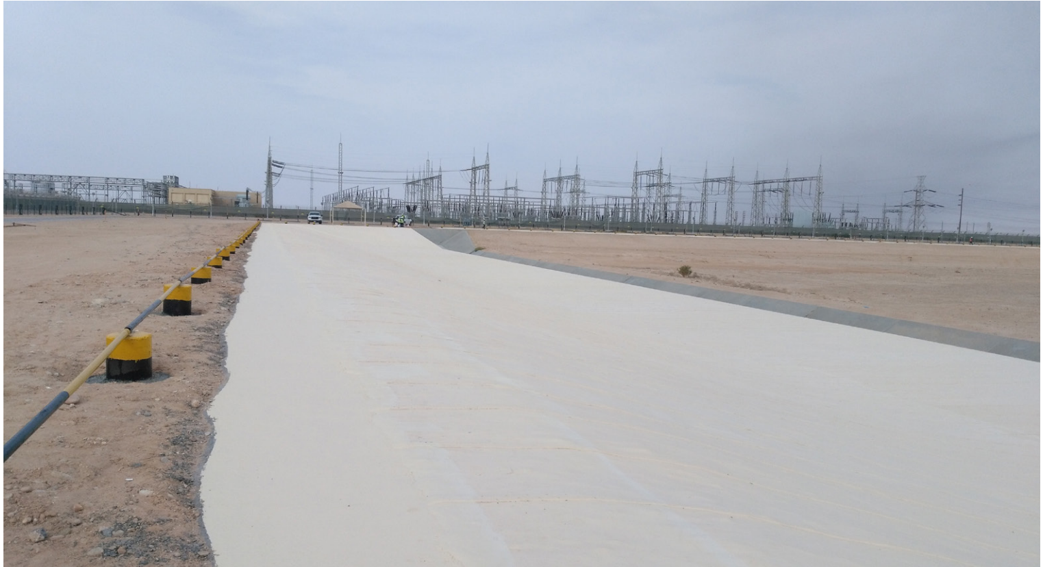
CC was painted once set to help the material blend in with surroundings
