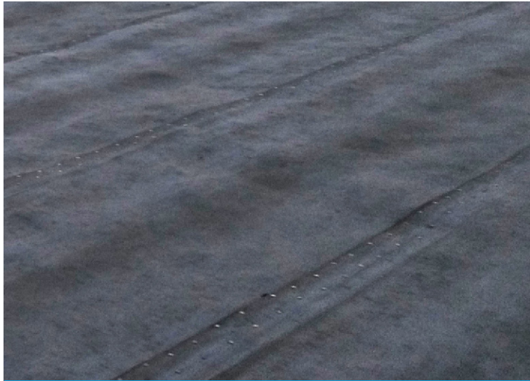
Screw jointed overlaps
