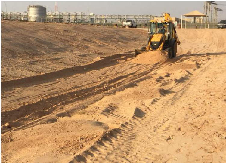
Stones and loose sand removed
