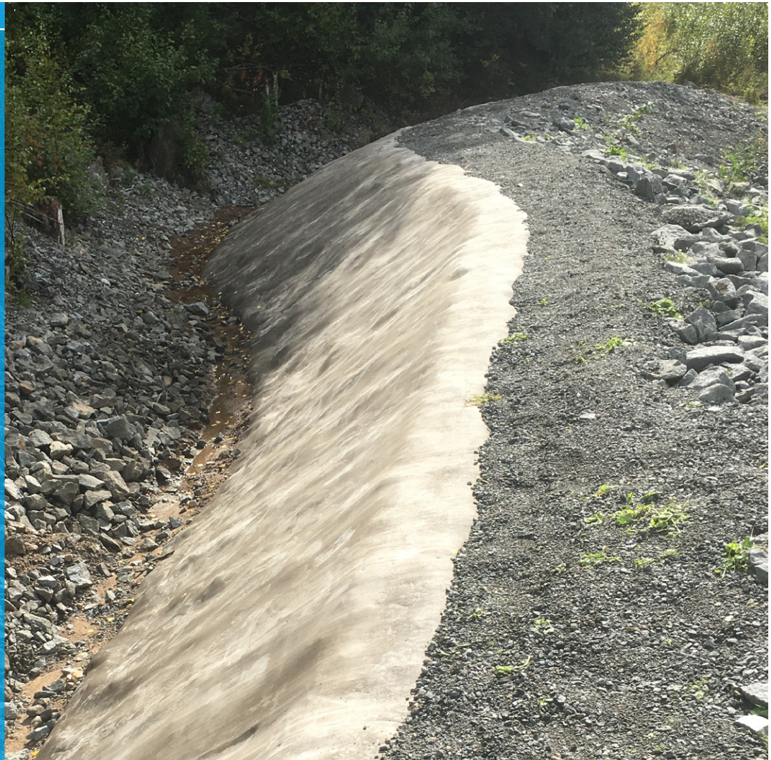
Completed slope protection installation in Sweden
