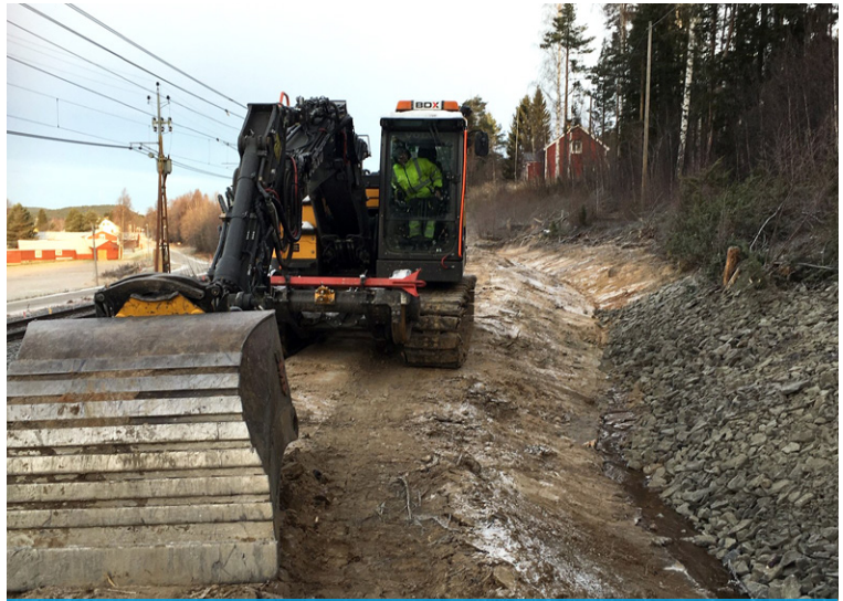
Vegetation, stones and rocks were removed and the substrate regraded
