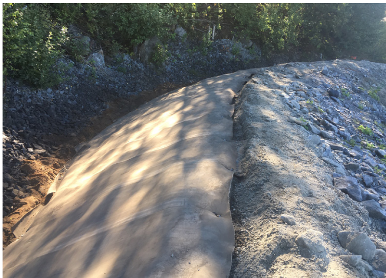
CC laid vertically down the slope face and secured in anchor trenches
