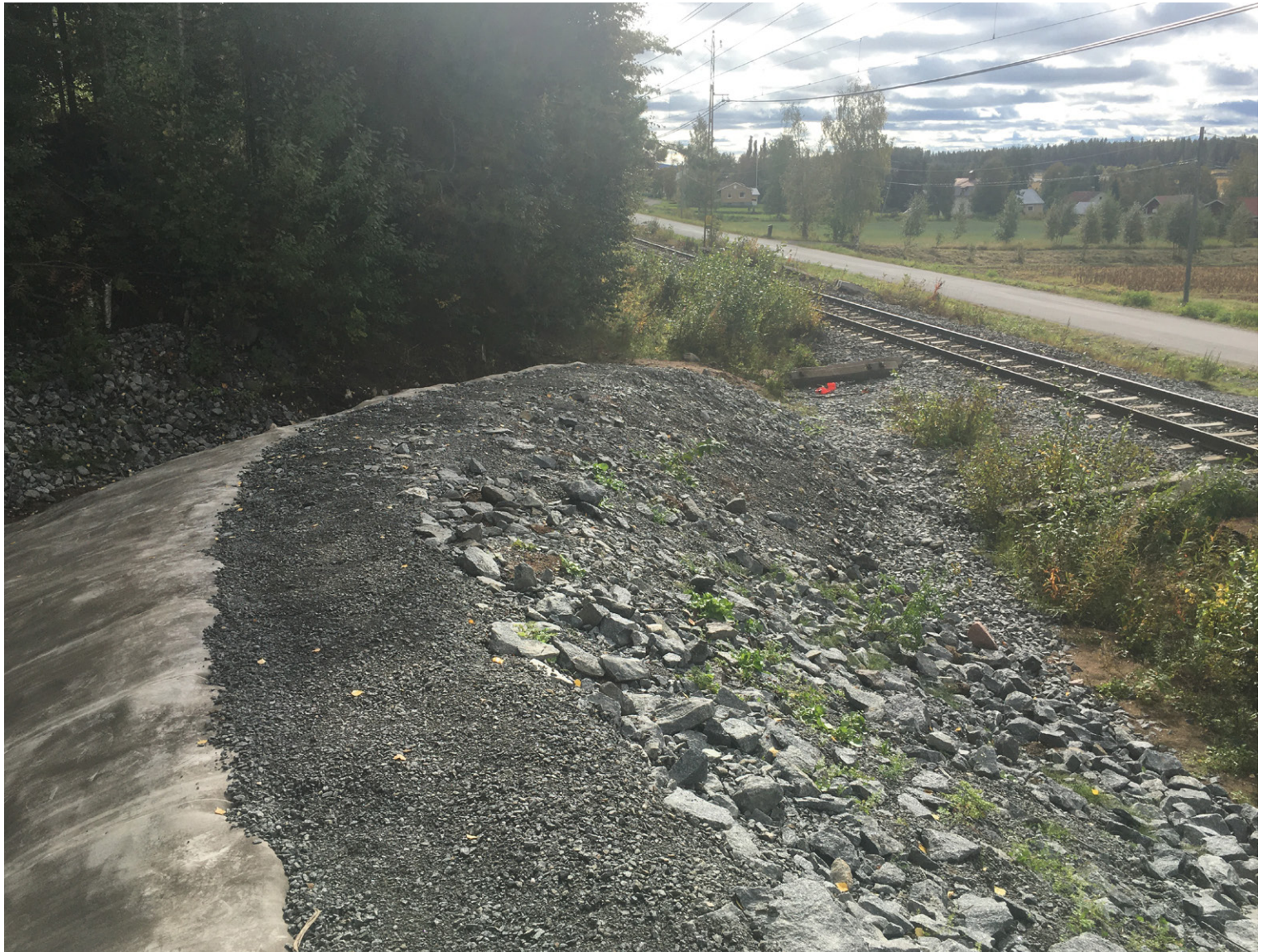
Anchor trenches backfilled for a neat termination; works carried out on a difficult to access site alongside a rail track
