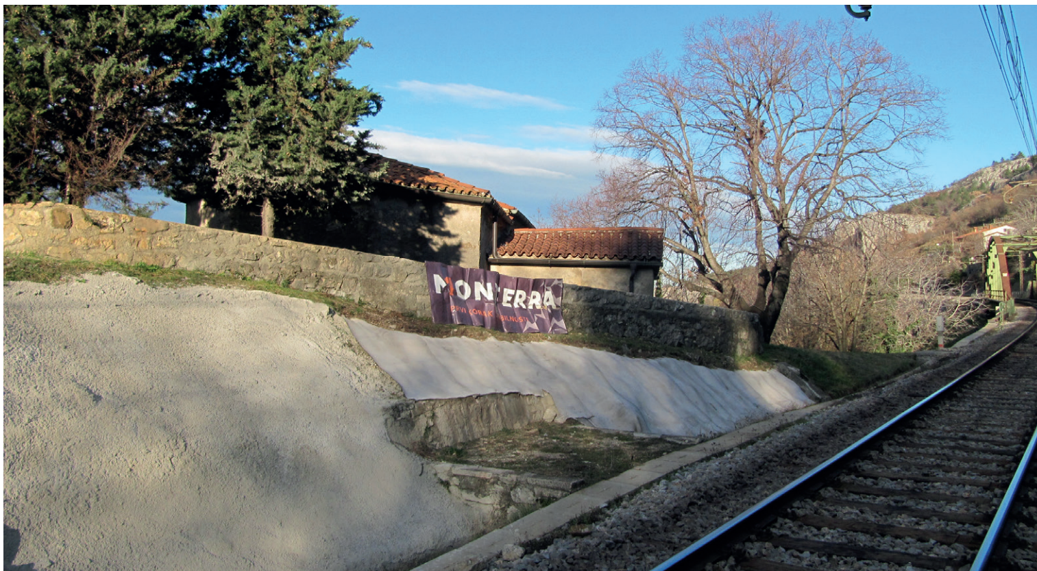
CC butted up to previous shotcrete installation
