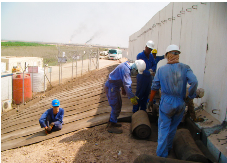
CC8™ lengths unrolled down the slope
