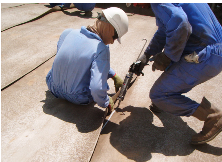
CT1 sealant applied to overlaps
