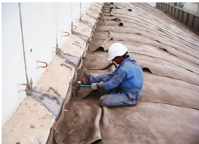
Masonry fixings and ground pegs
