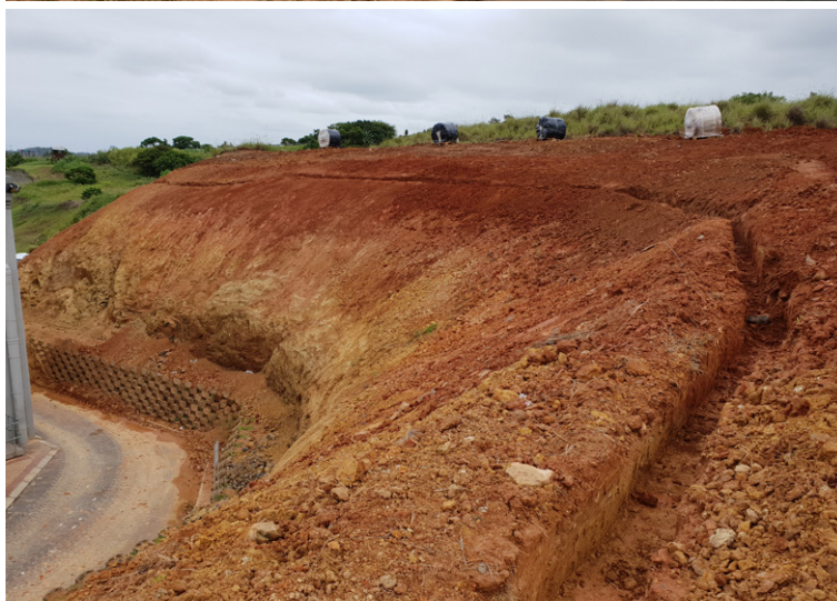
Anchor trenches were prepared at the crest
