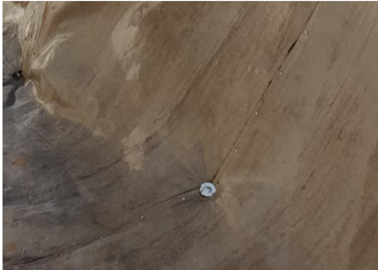
Round head pegs were used to secure CC to the slope face
