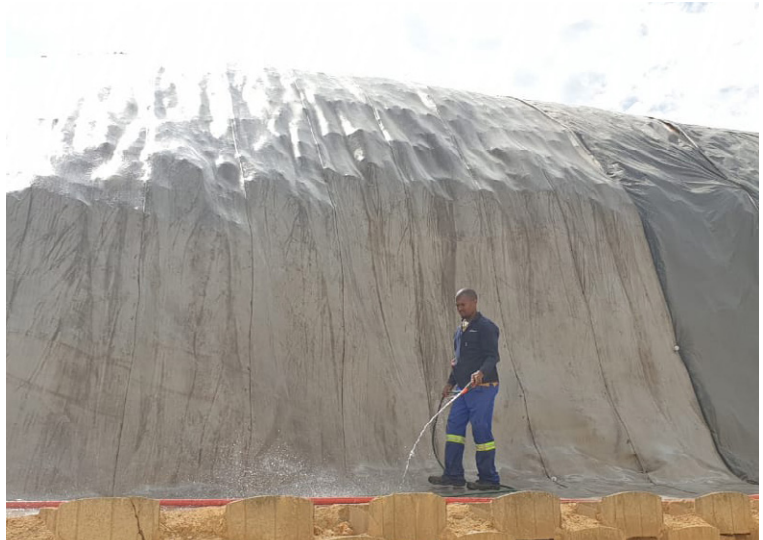
Hydration was given three times to ensure saturation in the hot conditions
