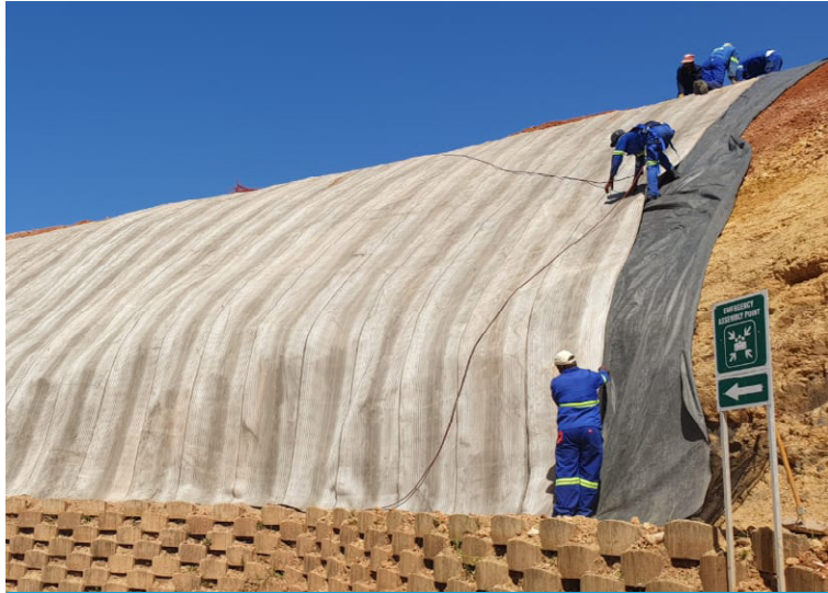
CC was laid over a geotextile layer which acted as a filtration layer
