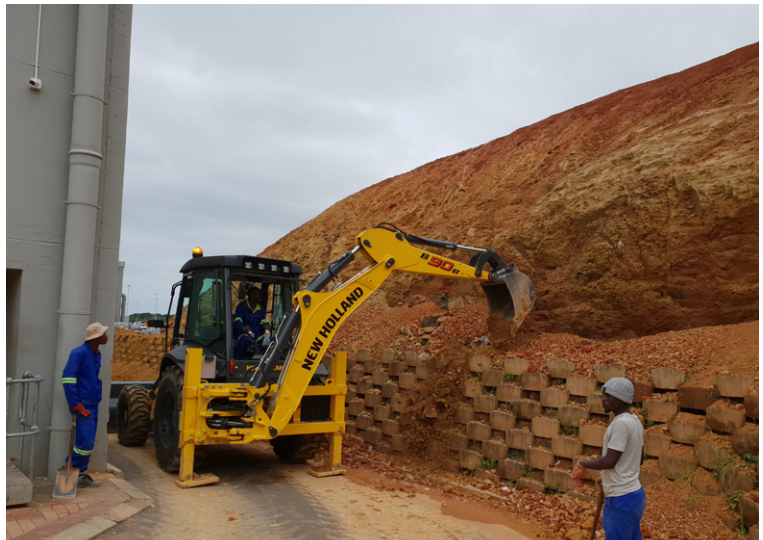
Slope face was trimmed for a smoother profile
