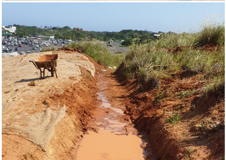
Cut-off drain prepared between cutting and natural ground level
