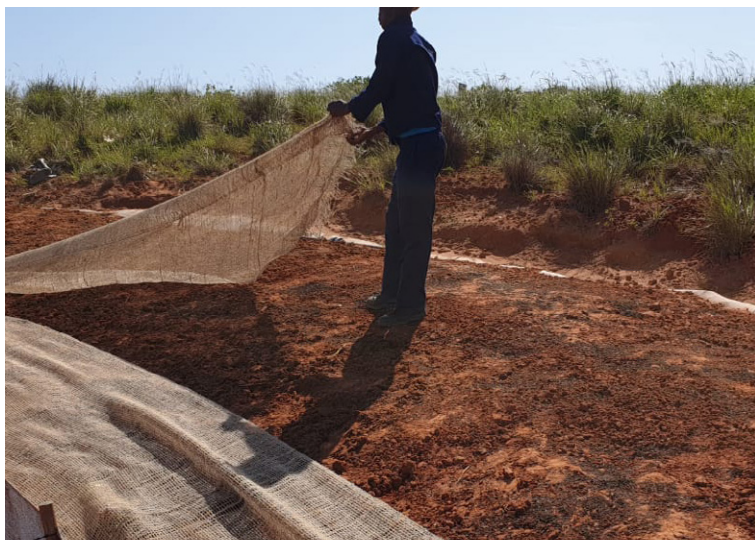
A vegetation mat was laid at the top of the slope to encourage regrowth
