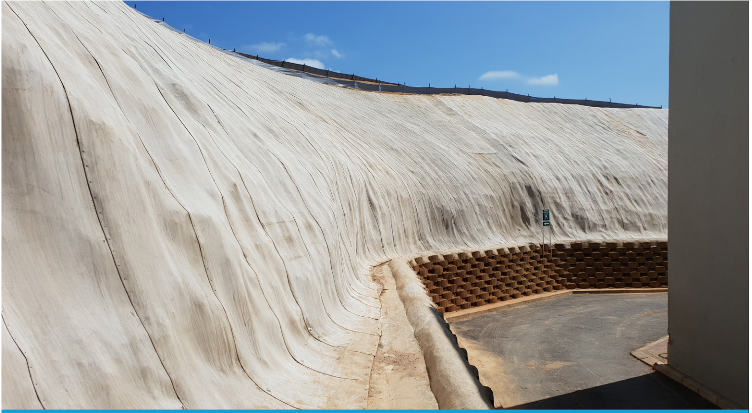
Completed CC slope protection installation in Shelly Beach, South Africa
