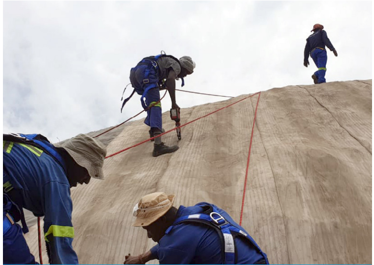
Overlapping CC layers were thermally bonded and screwed
