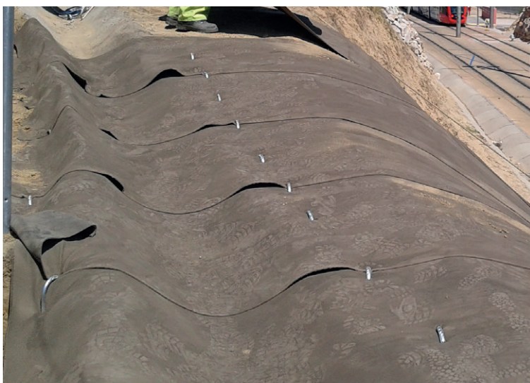
Pegs inserted every 500mm prior to screwing
