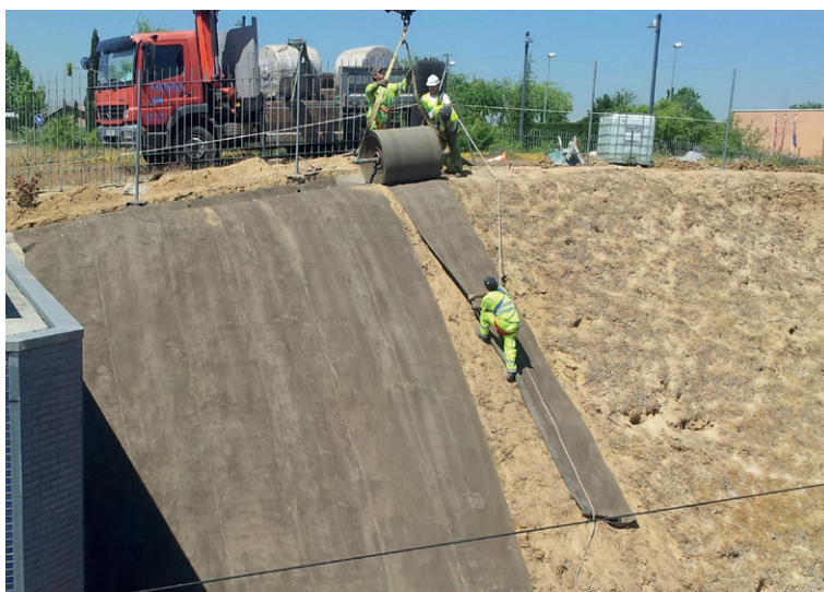
CC5™ spooled down slope
