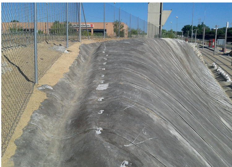
Backfilled anchor trench and drainage channel
