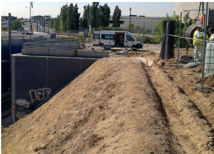
Prepared slope, drainage channel and anchor trench
