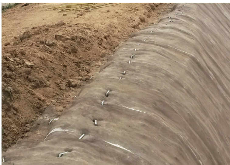
Ground pegs and anchor trench
