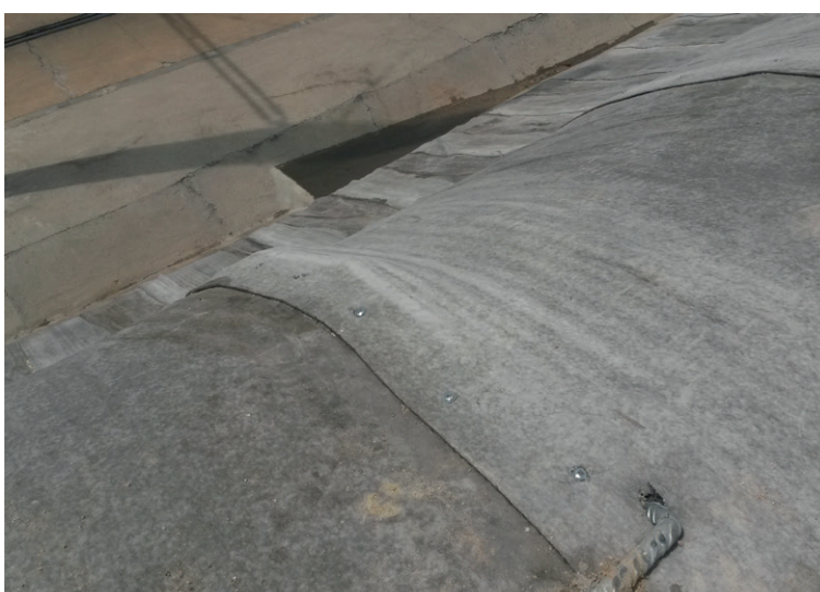
Screws inserted every 200mm
