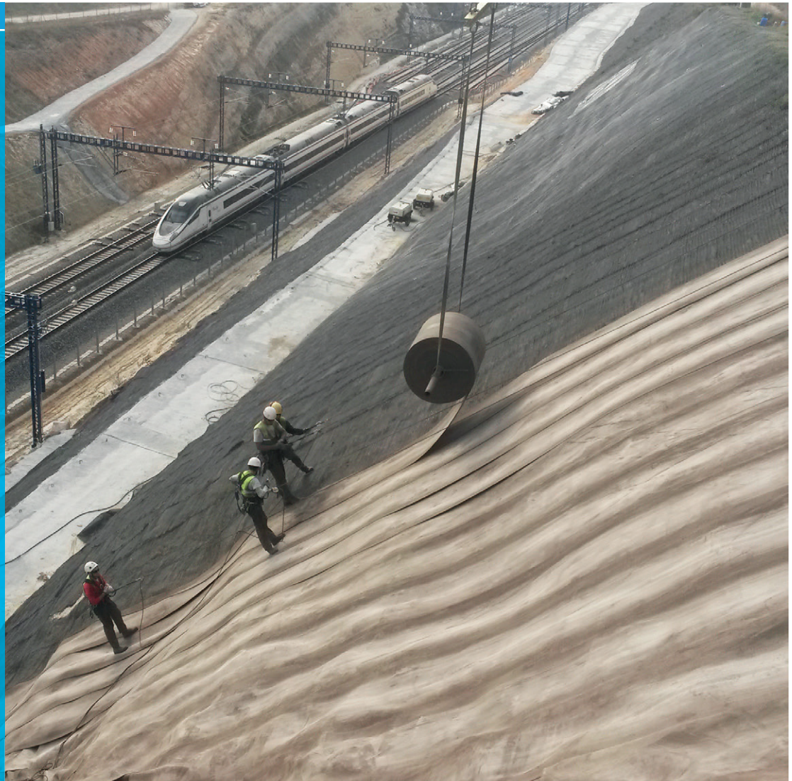
Deploying bulk roll of CC5™
