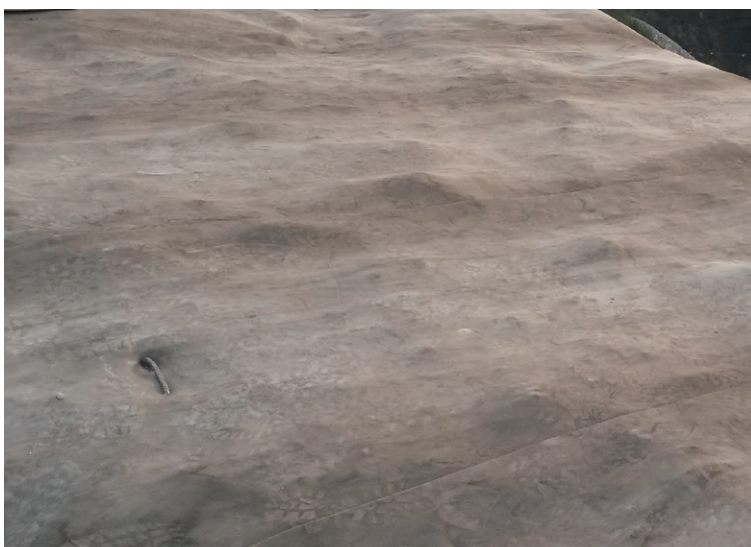
Ground pegs used to fix CC to substrate at crest
