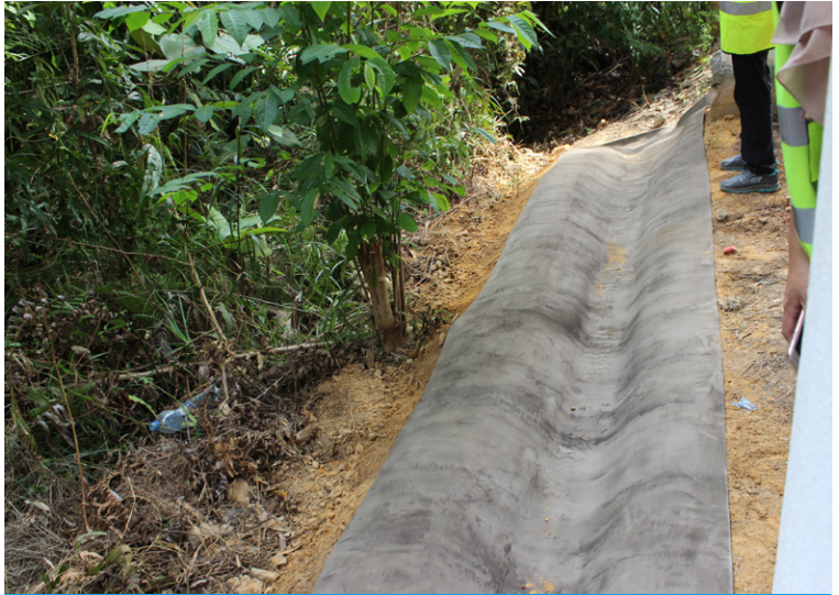
Installing CC within the drain at the side of the slope
