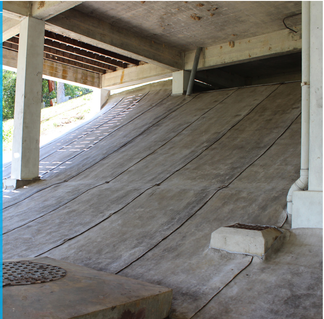
Completed slope protection installation
