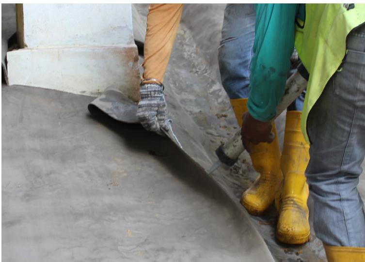
Applying sealant
