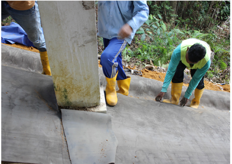
Cutting CC to accomodate existing concrete columns
