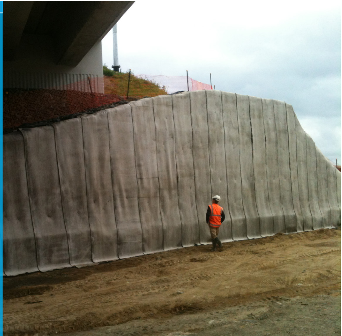
Completed section of slope lined with CC5
