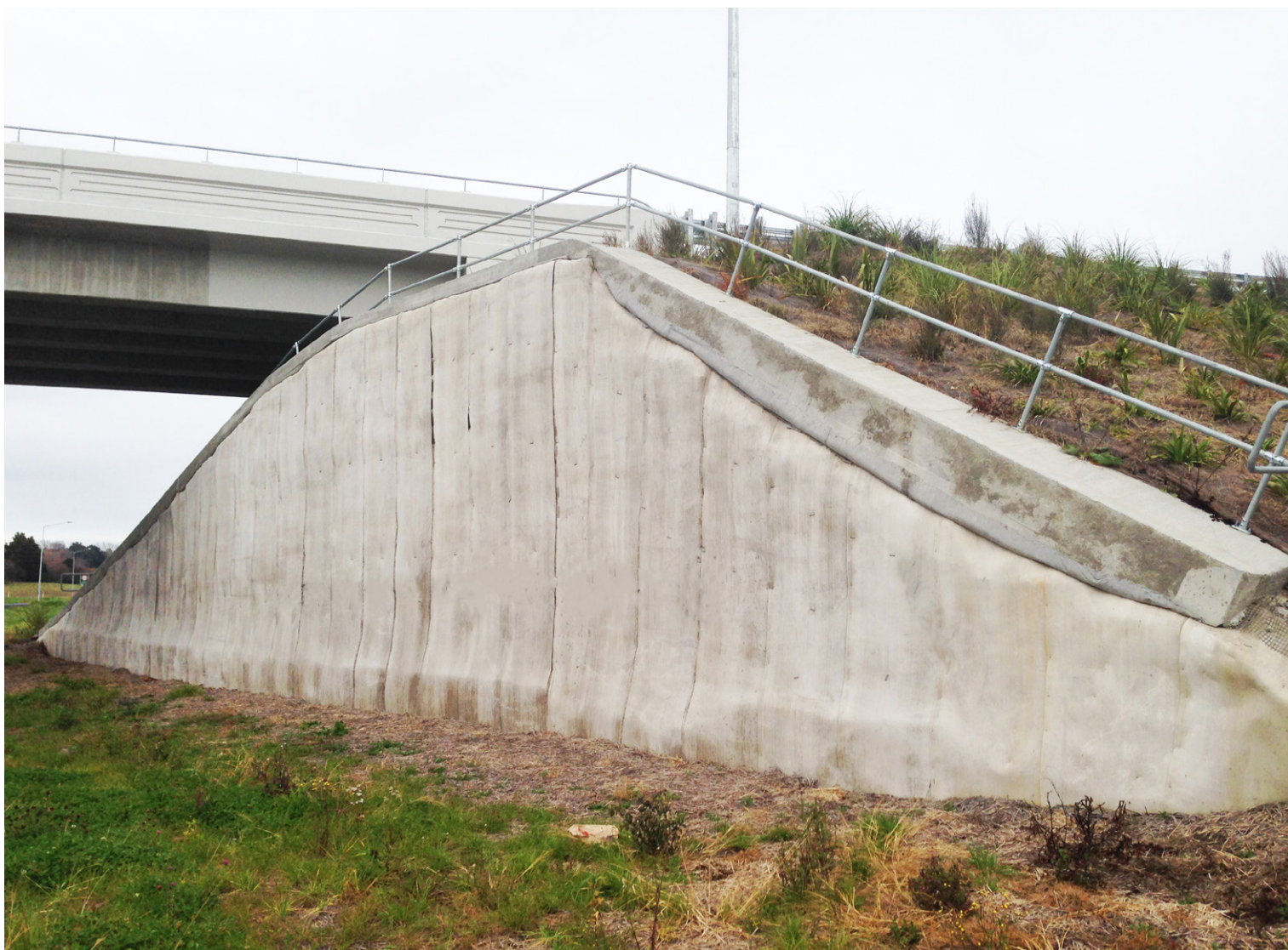
Completed CC slope three years after installation
