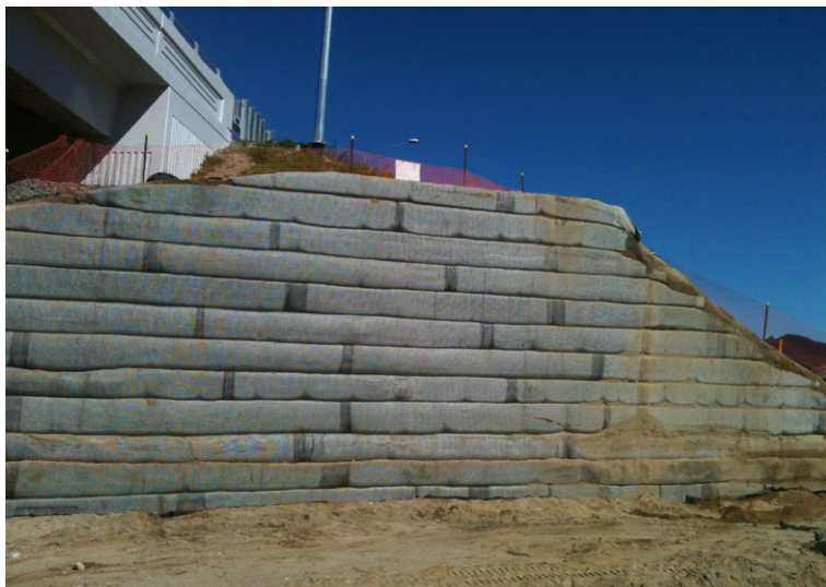
The abutment had been prepared with a geogrid prior to installation of CC
