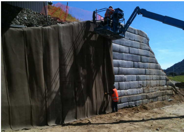
CC5 was cut to length on site to match the varying height of the abutment
