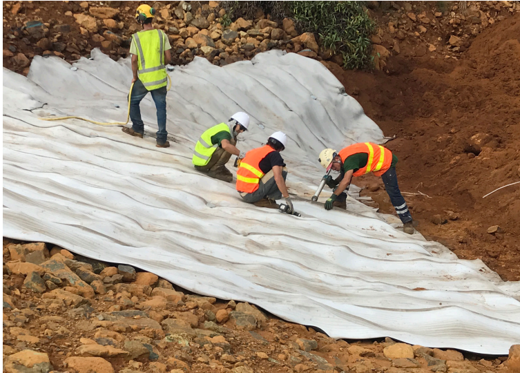
Installation - applying sealant to joints
