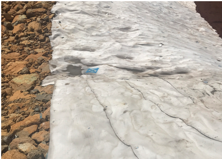
Close-up of completed CC installation
