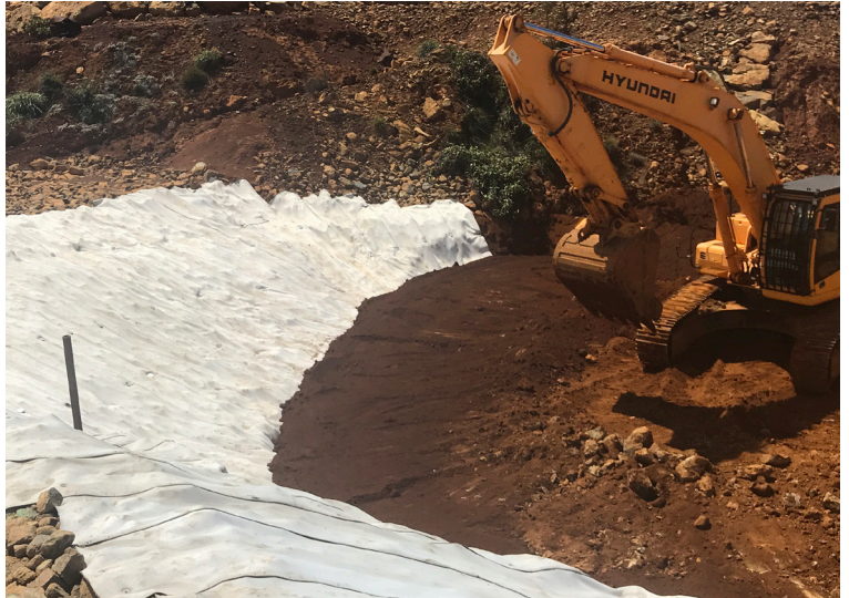
Burying edges of CC at toe of slope using excavator
