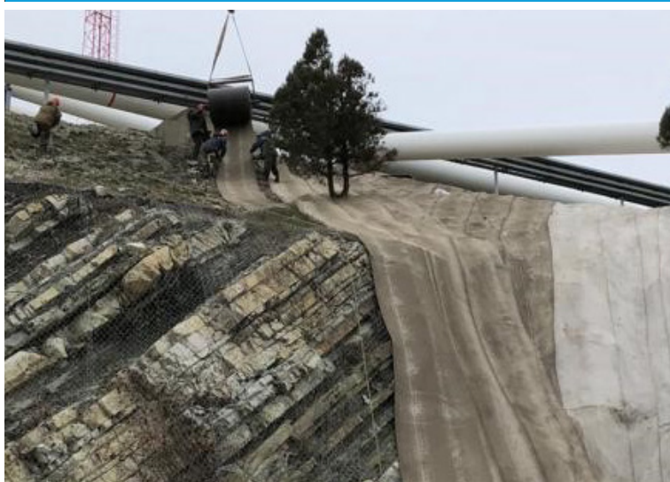
CC deployed from spreader beam
