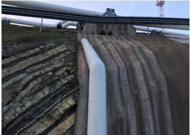
CC fitted around and underneath pipework
