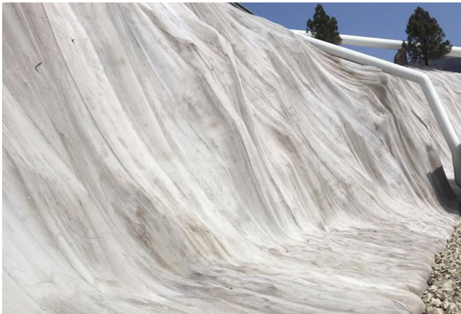
CC's flexibility allowed for easy accommodation of the slope's rocky surface
