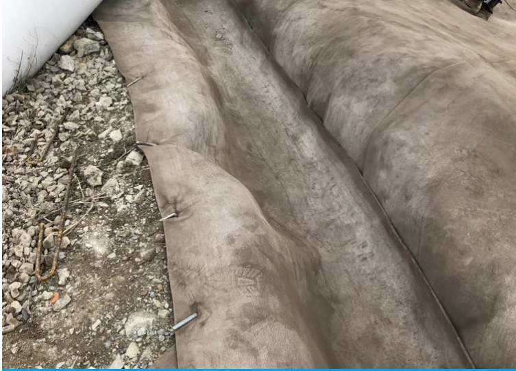
CC edges pegged at crest
