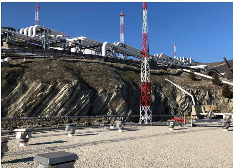
Rocky surface requiring protection
