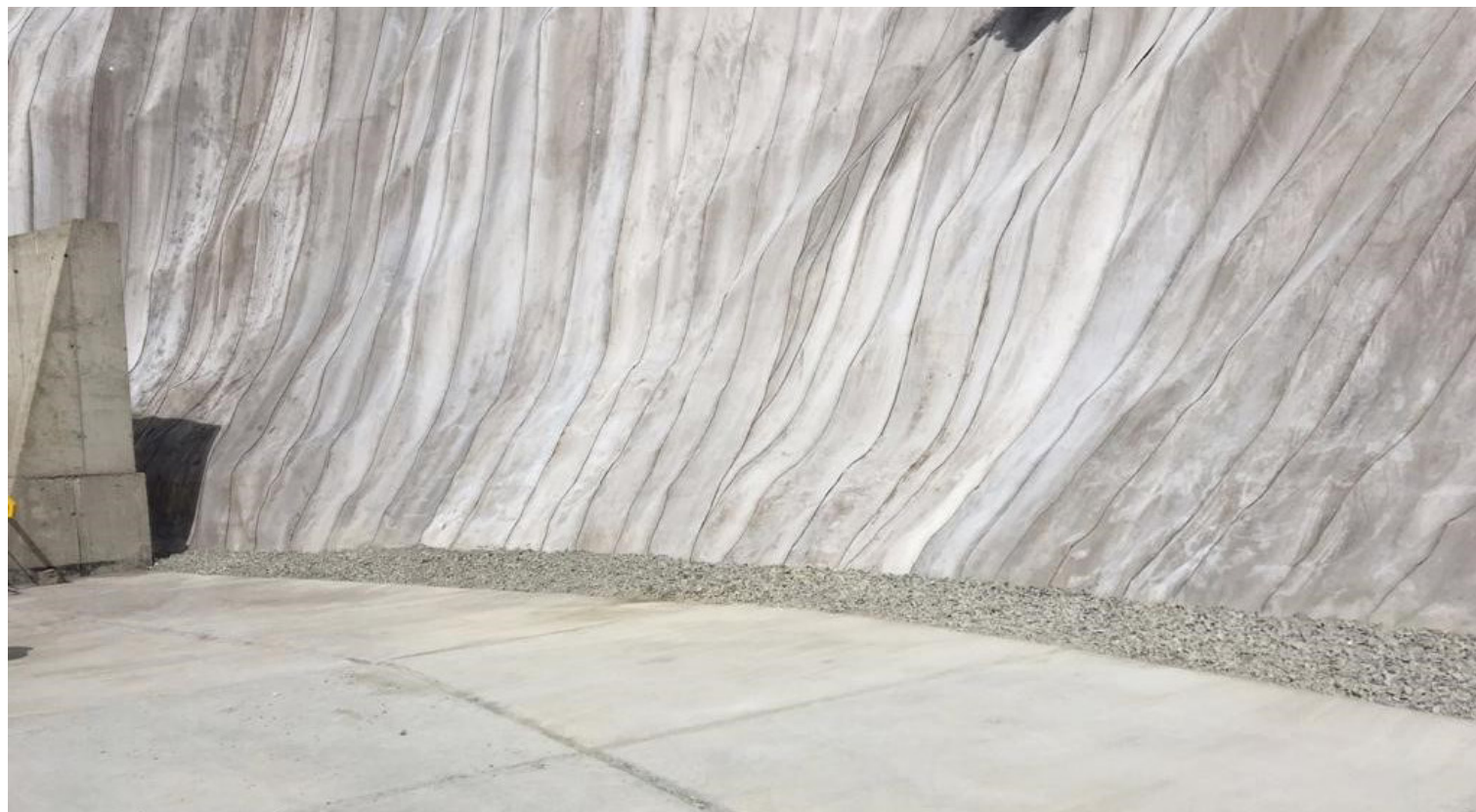
Lower section of completed slope and backfilled anchor trench
