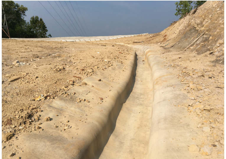
Small drainage channel created and lined for runoff management
