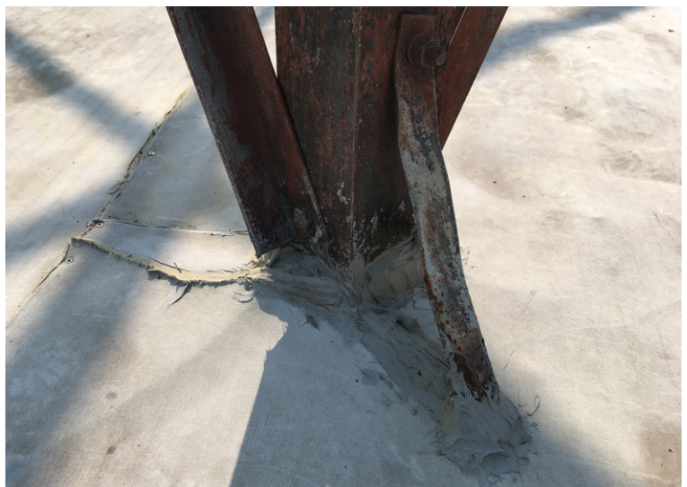
CC was easily installed around the pylon
