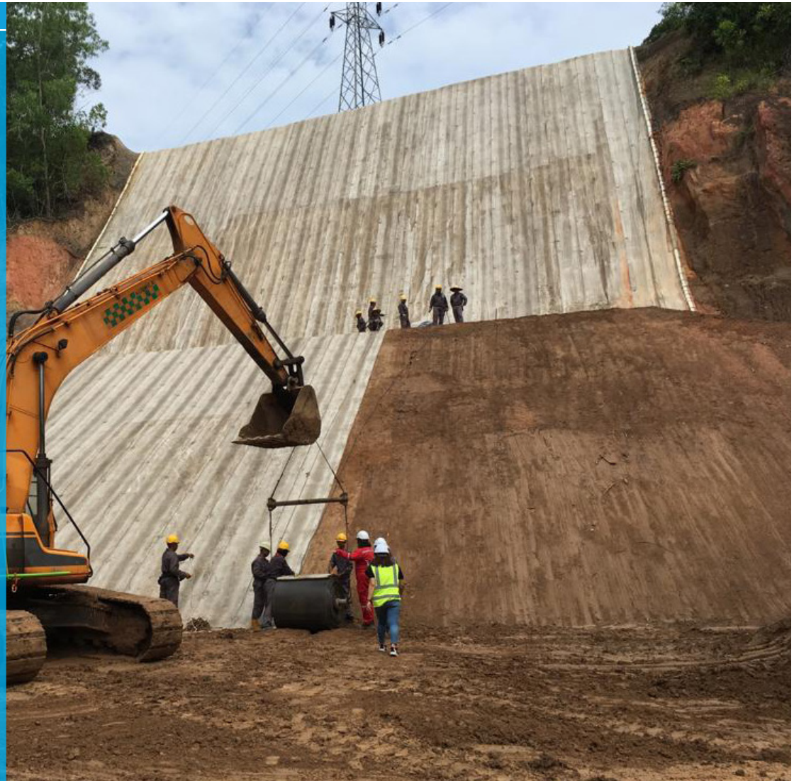
Installation of CC as slope protection solution in Brunei
