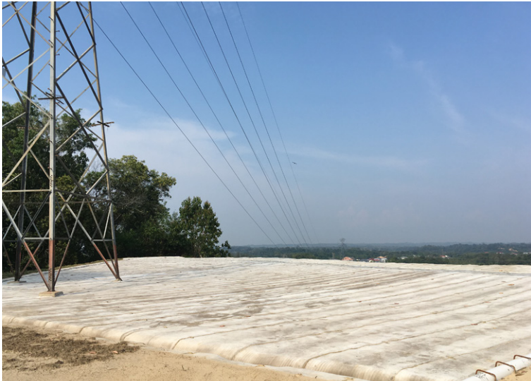
CC was also installed around the pylon
