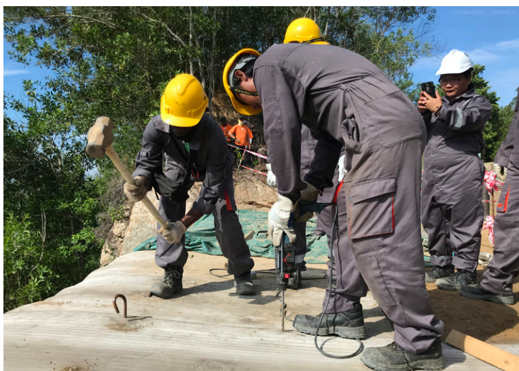
Fixing CC to ground using steel pegs
