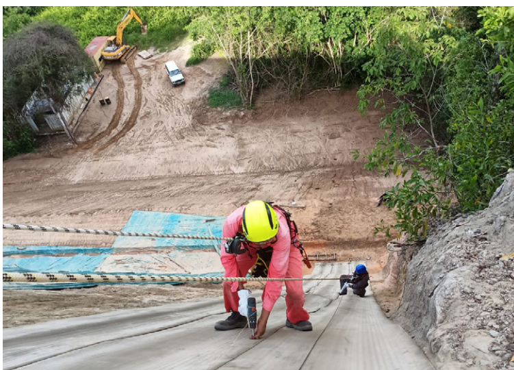
Screwing overlapped joints
