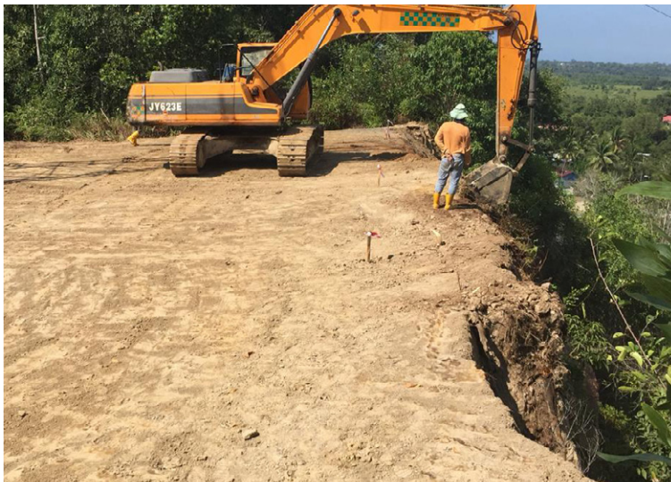
Removal of vegetation from crest of the slope
