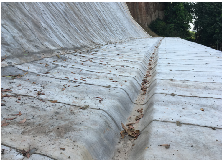
Lined step part way up slope - 2nd drain for further water management
