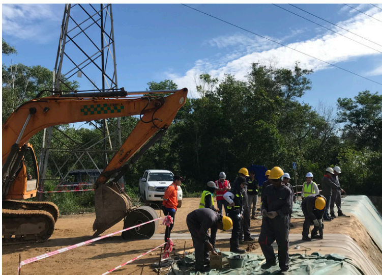
Deploying CC bulk roll for installation
