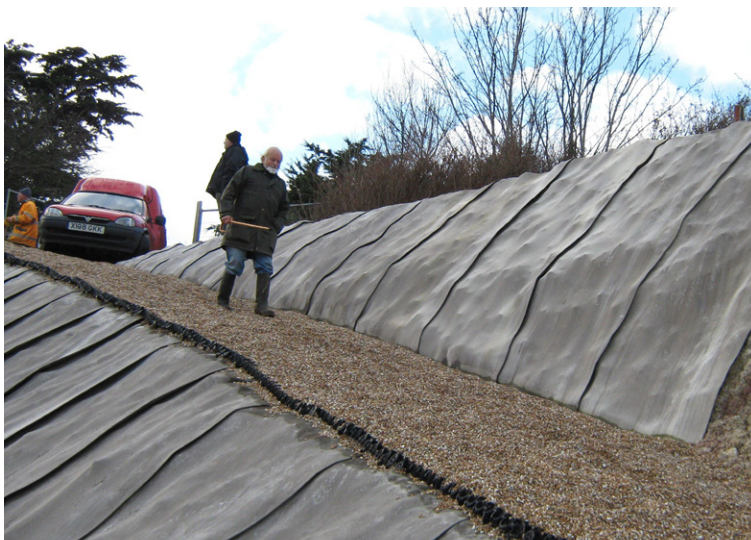
CC edges were buried following installation
