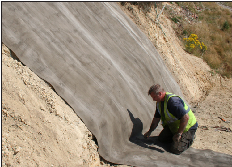
CC was fixed to substrate using ground pegs
