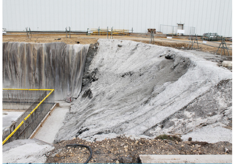
Previous protection measure with poured lean mix concrete
