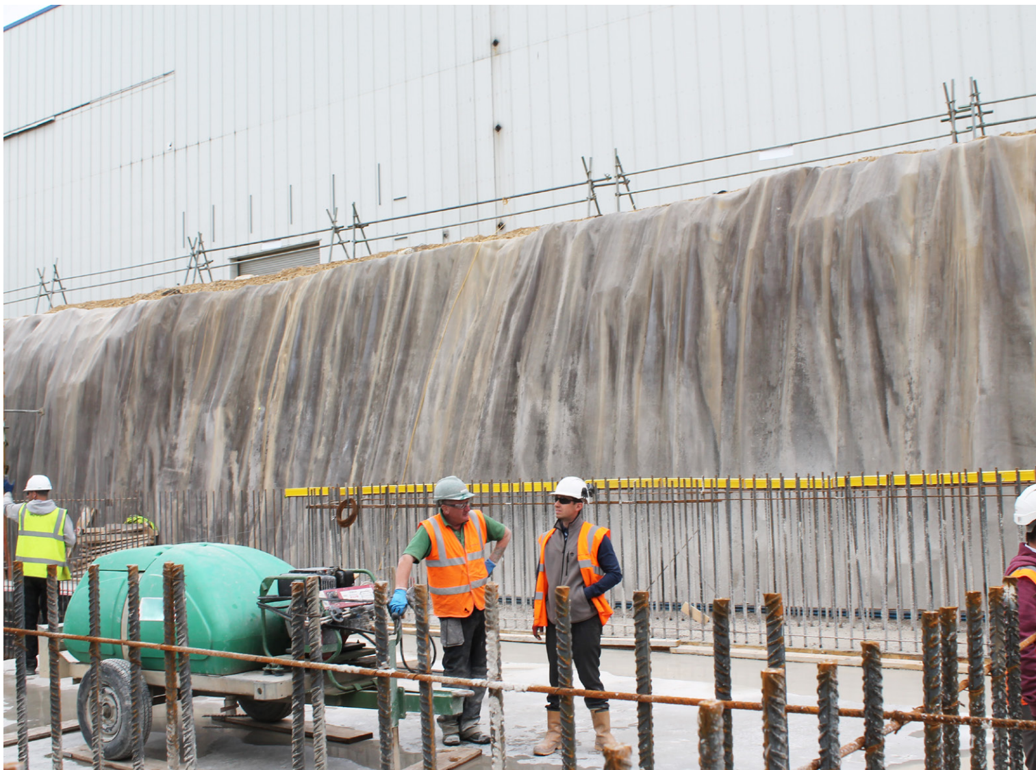
Completed CC lined north section of excavation
