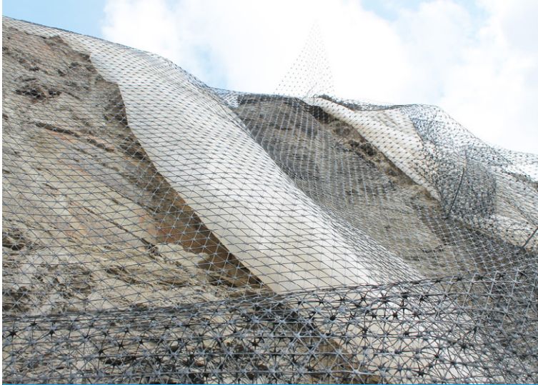
Previous protection measure with plastic sheeting and webbing
