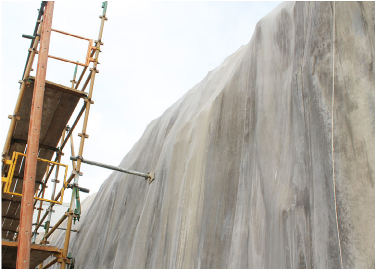
Previous protection measure with plastic sheeting and webbing
