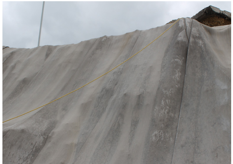
CC layers overlapped and screwed together
