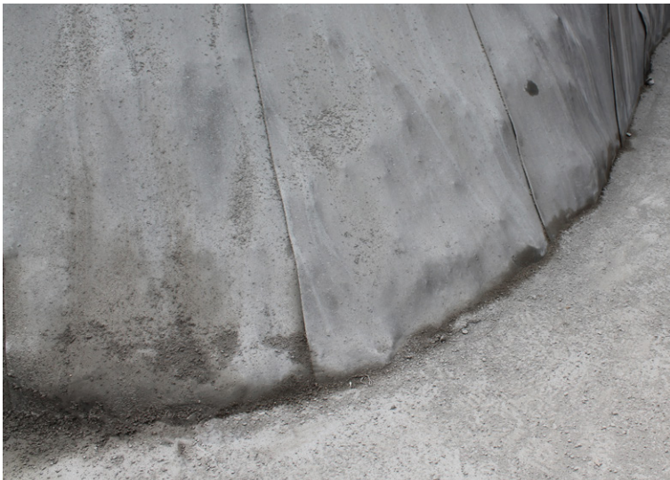
Poured concrete floor capture of CC ends
