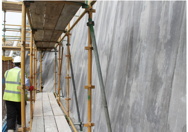
Scaffolding supported by CC lined rock face
