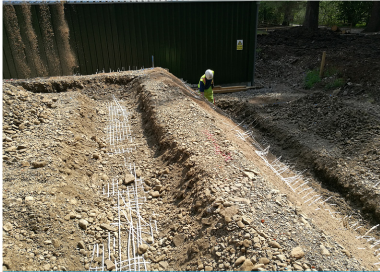
Bund reinforced using compacted soil and geogrids at 4500mm layers
