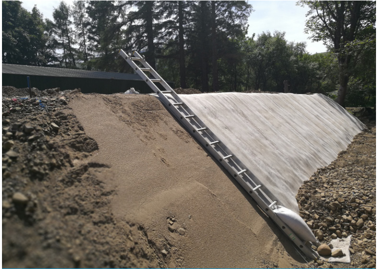
Sand compacted prior to CC installation
