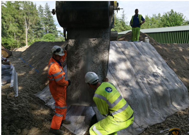
Deploying CC bulk roll
