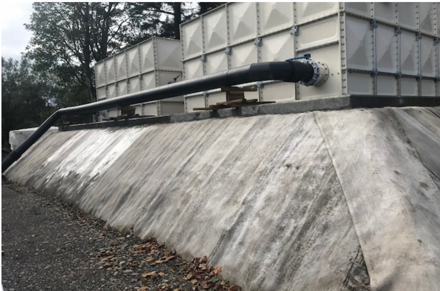
Concrete slab poured and header tanks and pipes installed after CC set
