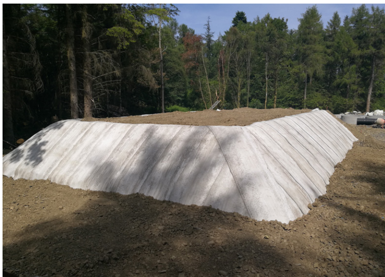
Backfilled anchor trenches and corner detail
