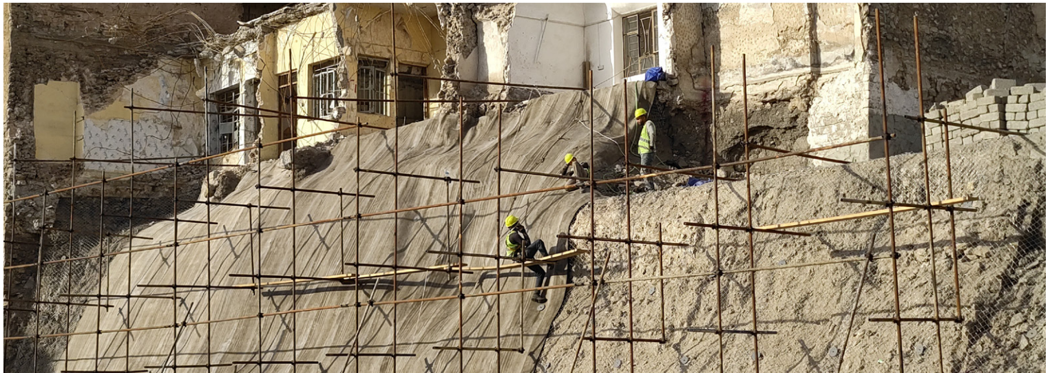
Steel mesh was installed under the CC
