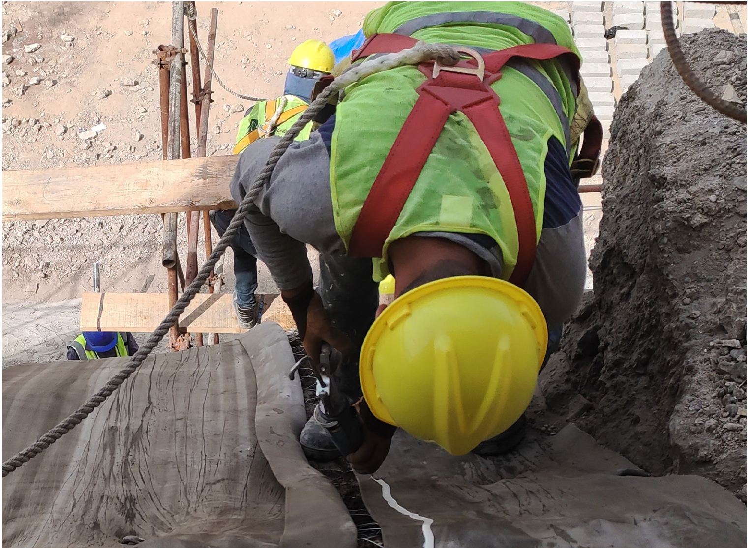
Using an adhesive sealant
