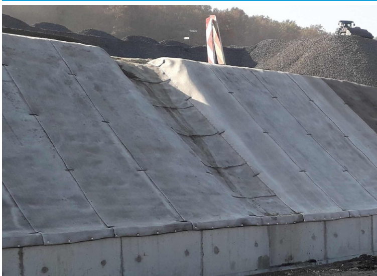
Section of transversely laid CC sections for surface runoff
