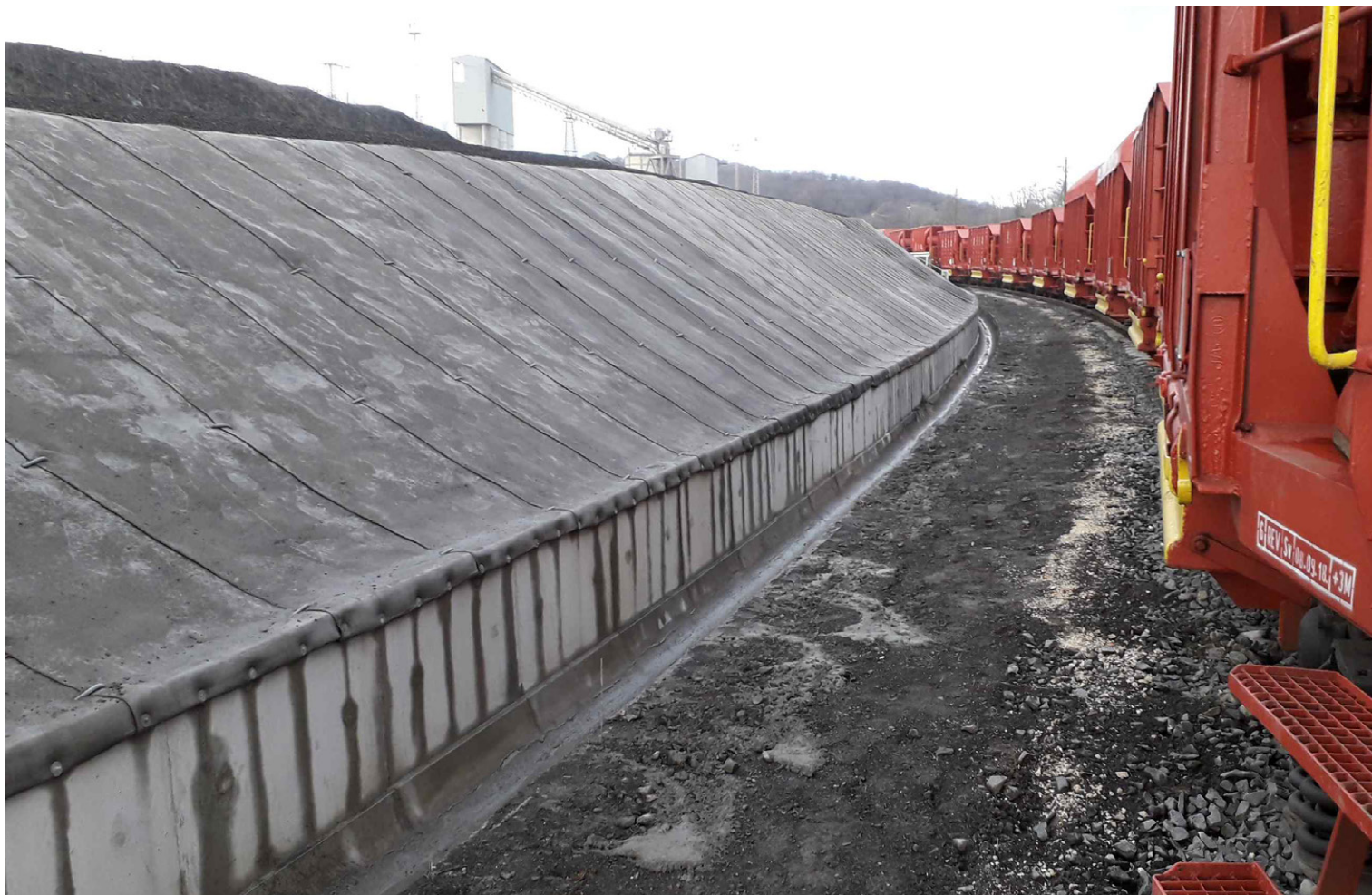
Completed section of CC slope protection installation
