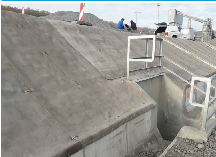
Termination detail onto concrete wall at slope toe
