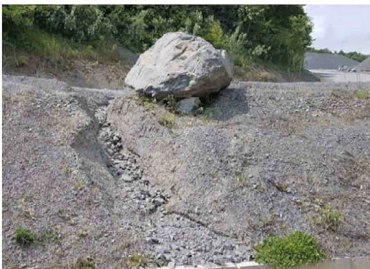
Scour of slope caused by erosion
