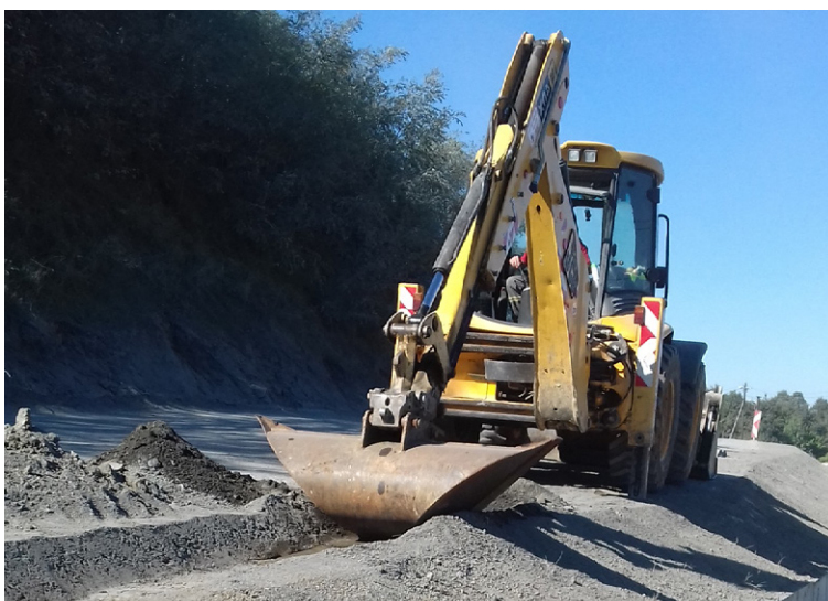
Anchor trenches created using digger and V-bucket
