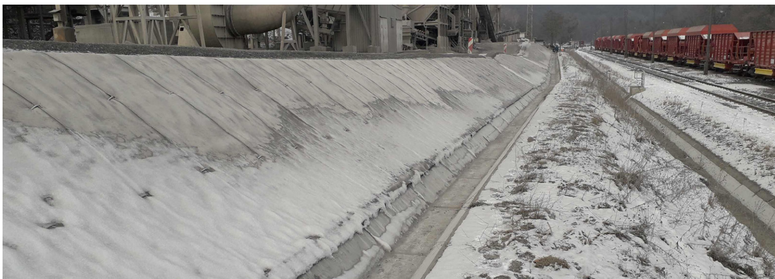
The CC slope is able to withstand freeze thaw conditions experienced during colder months in the area
