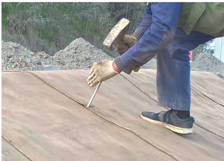
Ground pegs used to fix CC to substrate
