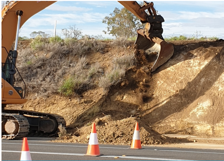
Removing vegetation with excavator
