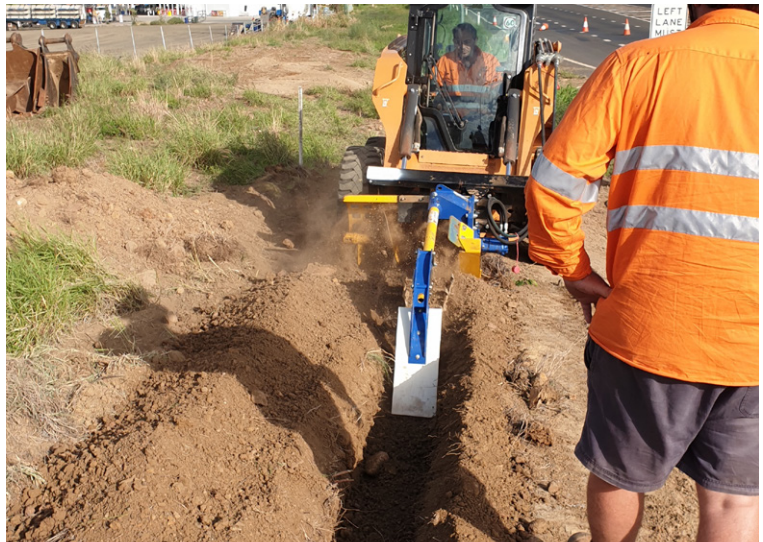
Digging anchor trenches at crest of slope
