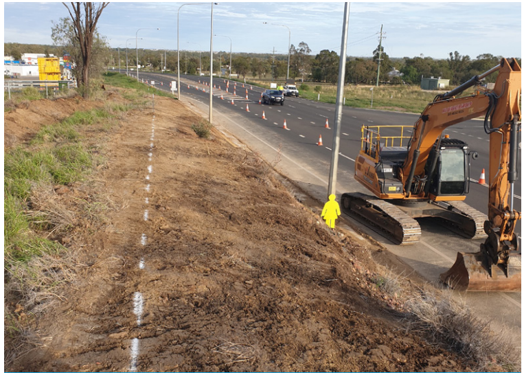
Anchor trench marked out following initial ground preparation
