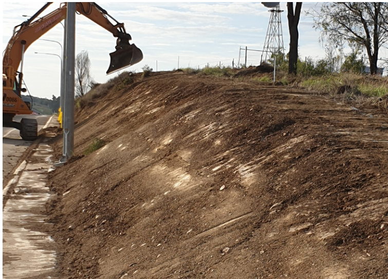
Grading the slope profile
