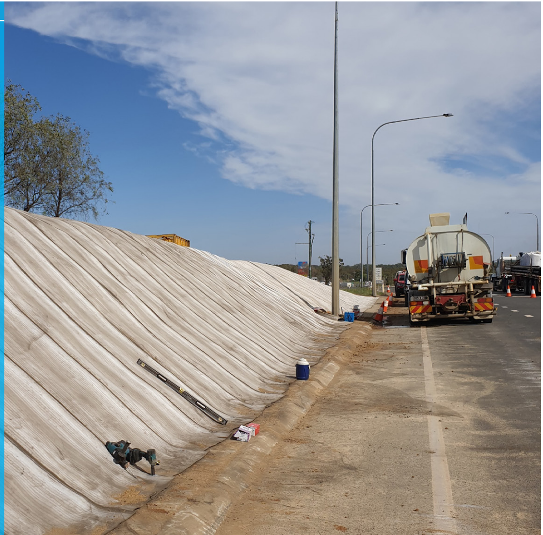
Completed slope protection installation alongside the Warrego Highway in Roma, Australia
