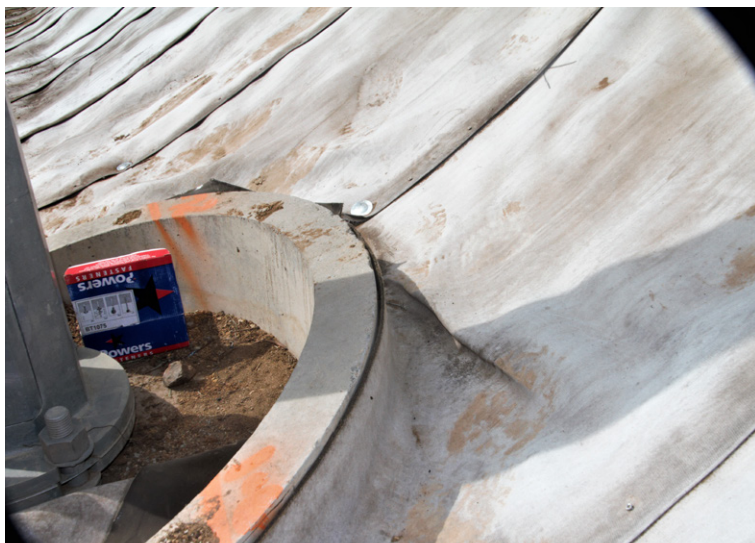
Termination around concrete kerb
