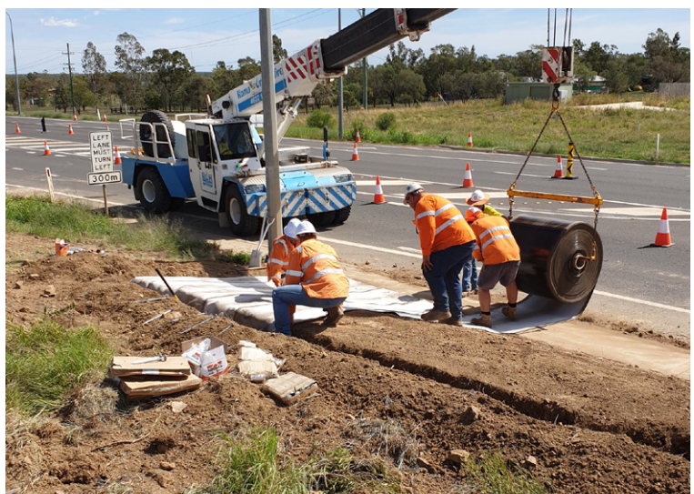
Securing CC within anchor trenches
