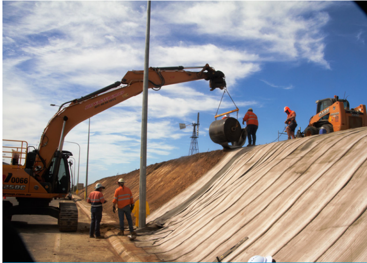
A spreader beam and plant made installation easier
