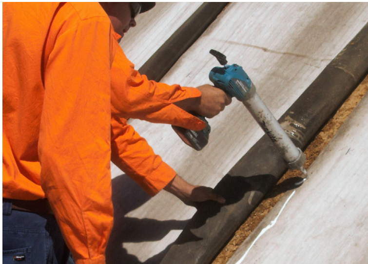
Sealant used to provide a low permeability joint
