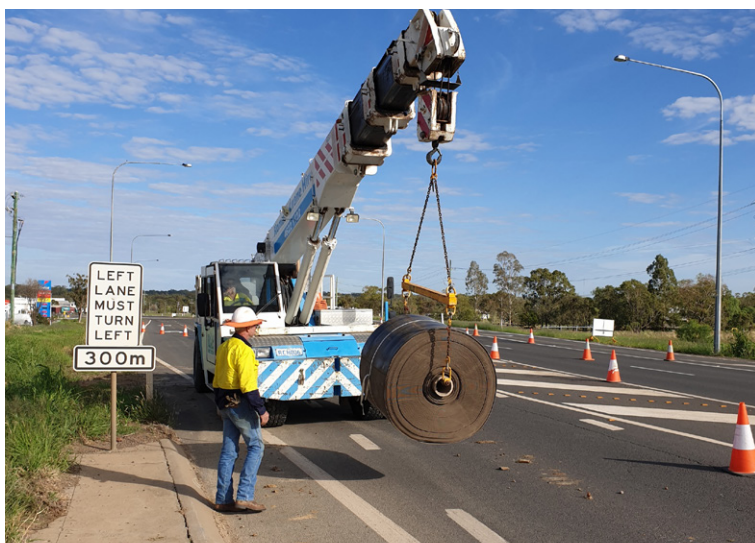
Mounting CC bulk rolls to spreader beam
