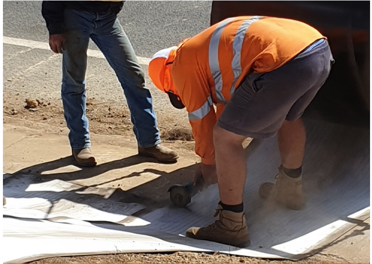
Cutting CC to length with a disc cutter
