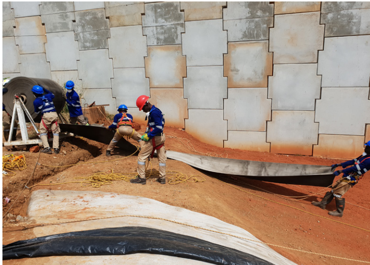
Deployment of CC bulk roll
