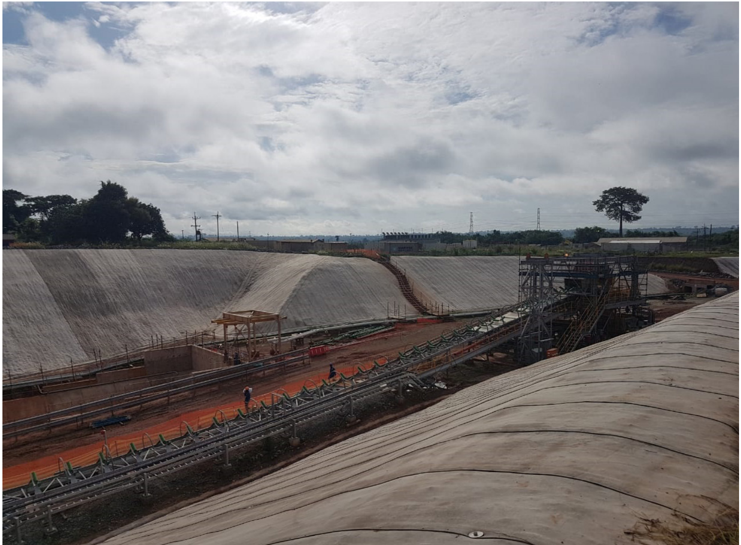
Completed CC lined slope sections
