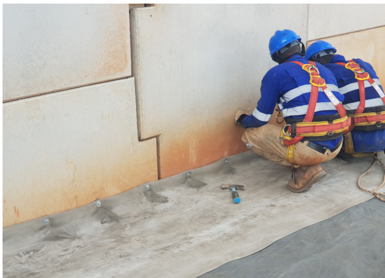
Termination of CC to existing wall
