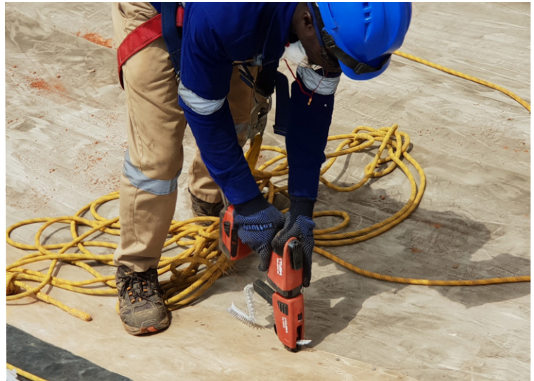
Joining CC overlaps with stainless steel screws
