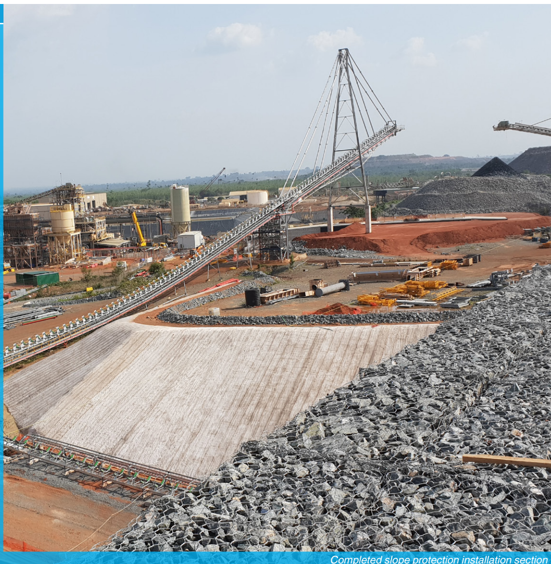
Completed slope protection installation section
