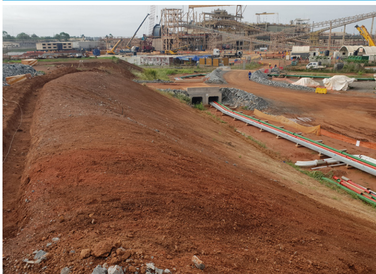
Slope section following ground preparation
