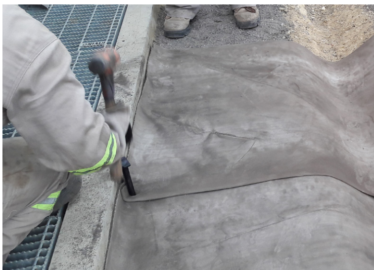
Securing CC to substrate using ground pegs
