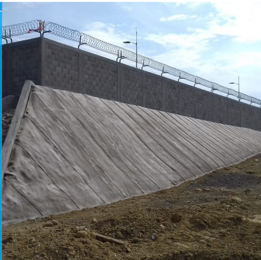
Completed slope section lined with CC
