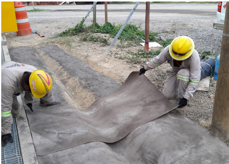
Laying pre-cut CC lengths
