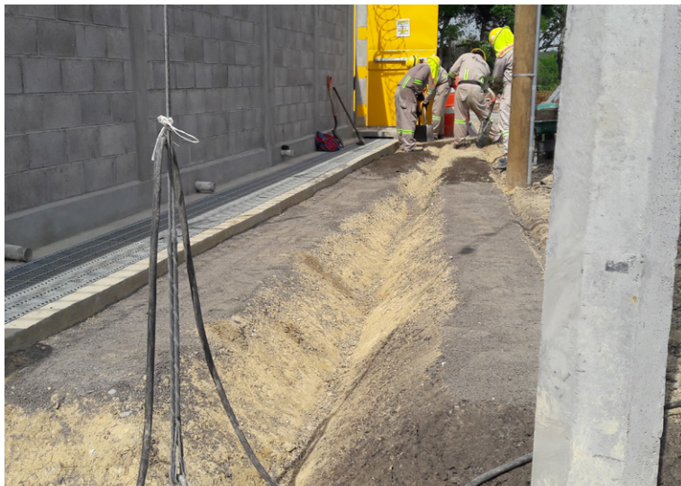
Channel following excavation and ground preparation
