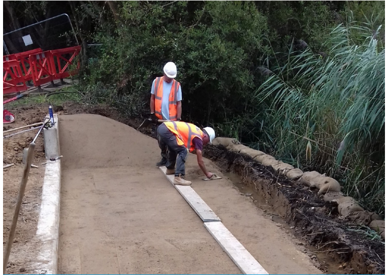
Compacted and troweled to smooth substrate
