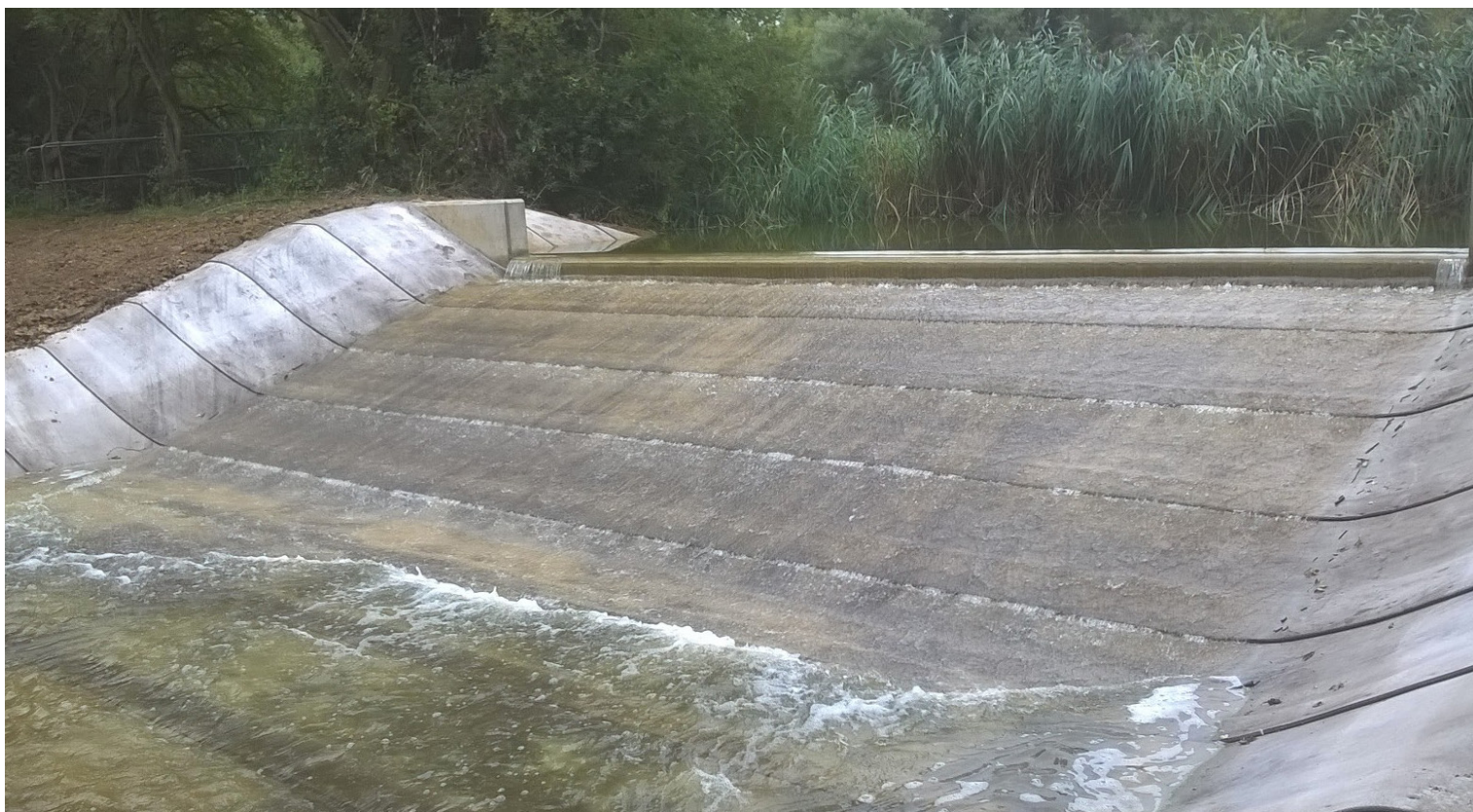
CC-lined spillway in use
