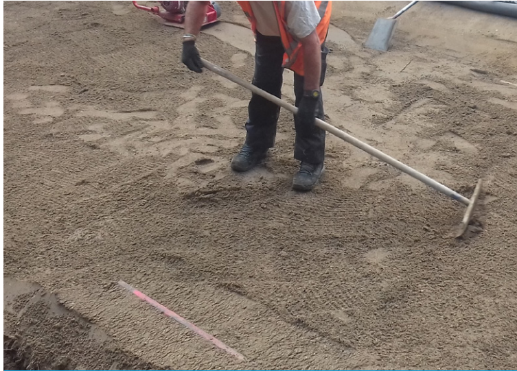
Sand raked then compacted to create smooth profile
