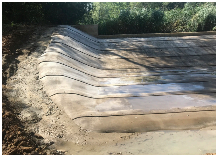
CC edges buried in anchor trenches with poured concrete
