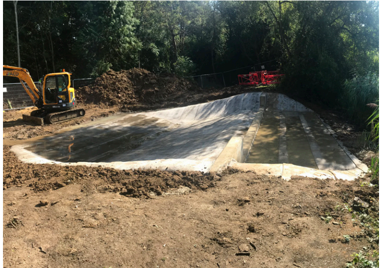
Spillway following CC installation
