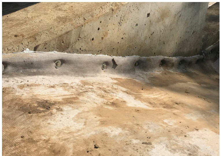
CC edges fixed to headwall using Hilti shot fired nails
