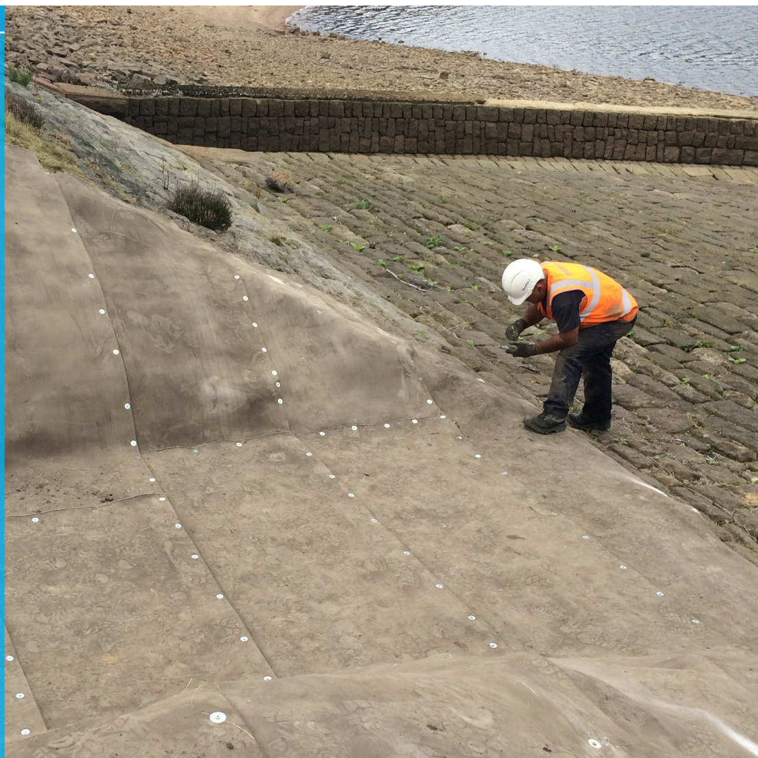
Drainage channel prior to hydration.
