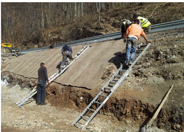
The CC was installed down the steepest section of the slope
