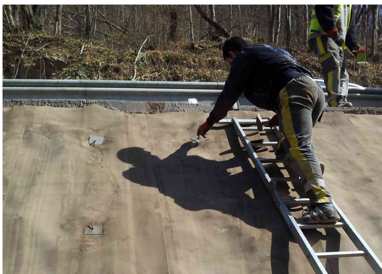
The CC was secured using ground pegs
