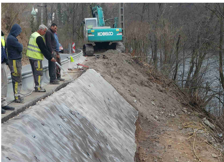
The CC was hydrated using a hose
