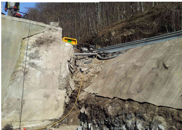
The remainder of the collapsed supporting wall
