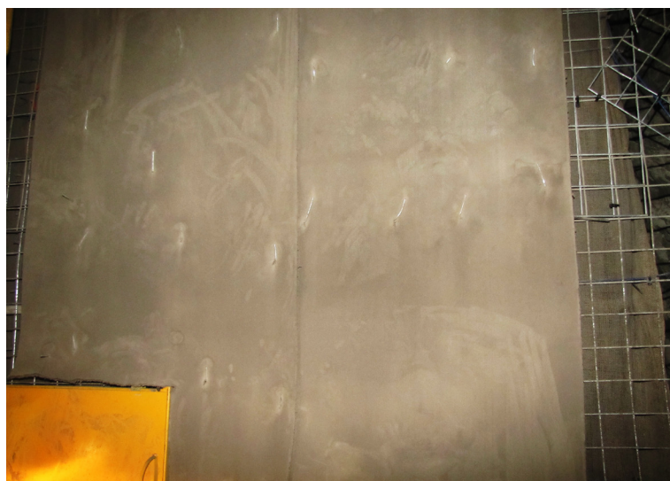
Prongs holding CC to mesh
