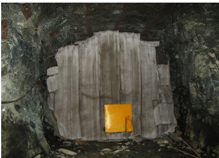
Finished vent wall installation
