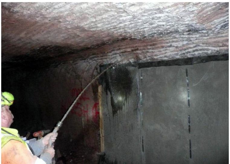
CC hydrated using on-site equipment
