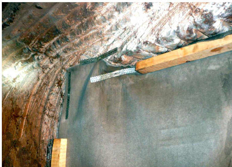
Battens, 200mm steel and screws used to provide strong fixing to rock
