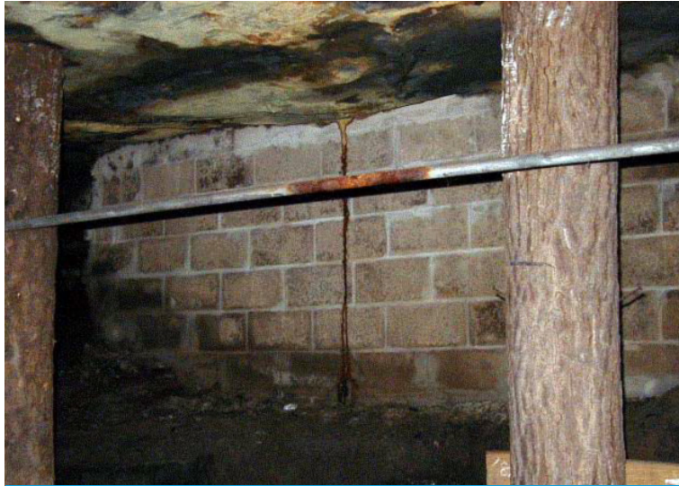
Concrete block vent walls had proved expensive and difficult to install
