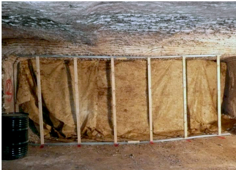
Frame created using British Gypsum branded aluminium stud wall system
