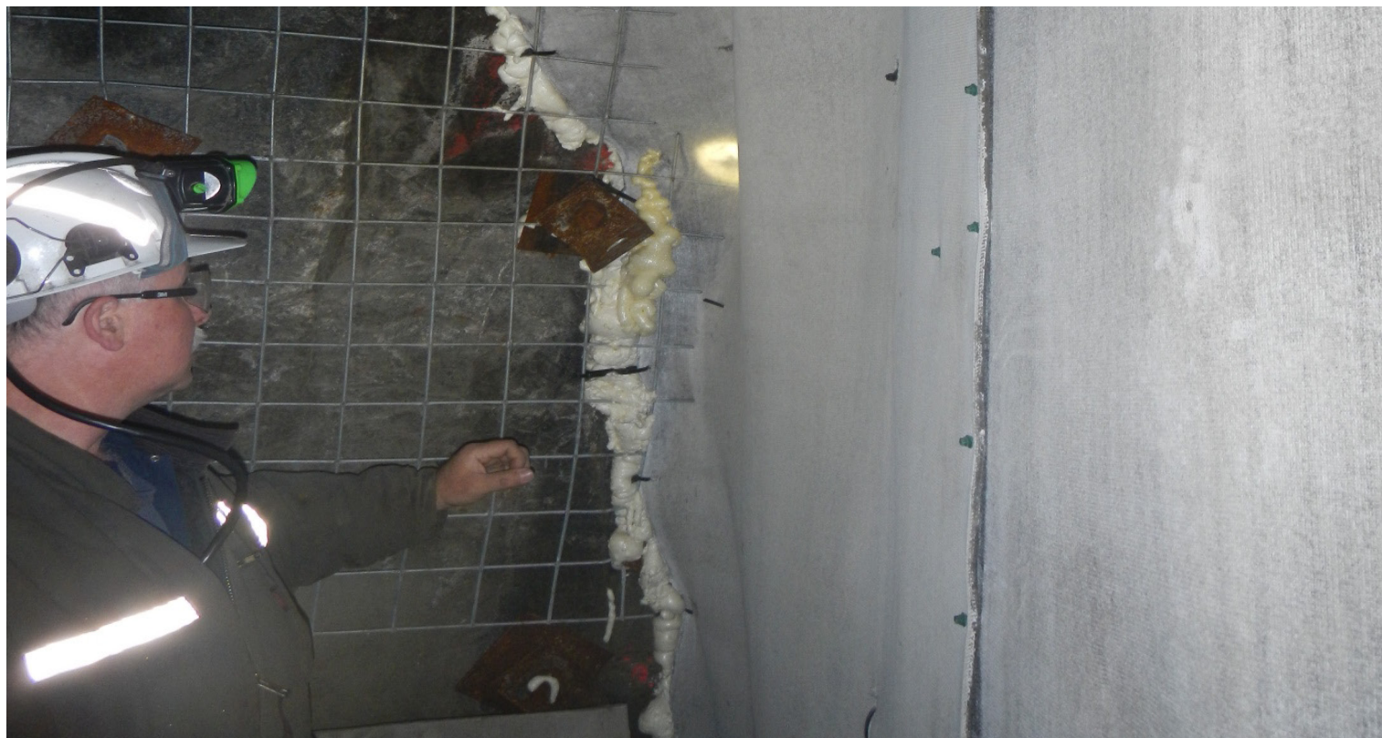
Spray foam used to fill any voids between vent wall and surrounding rock
