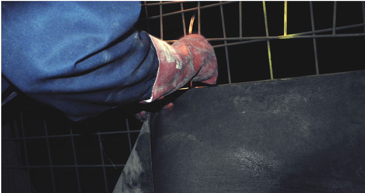
Industrial cable ties used to attach CC to wire frame
