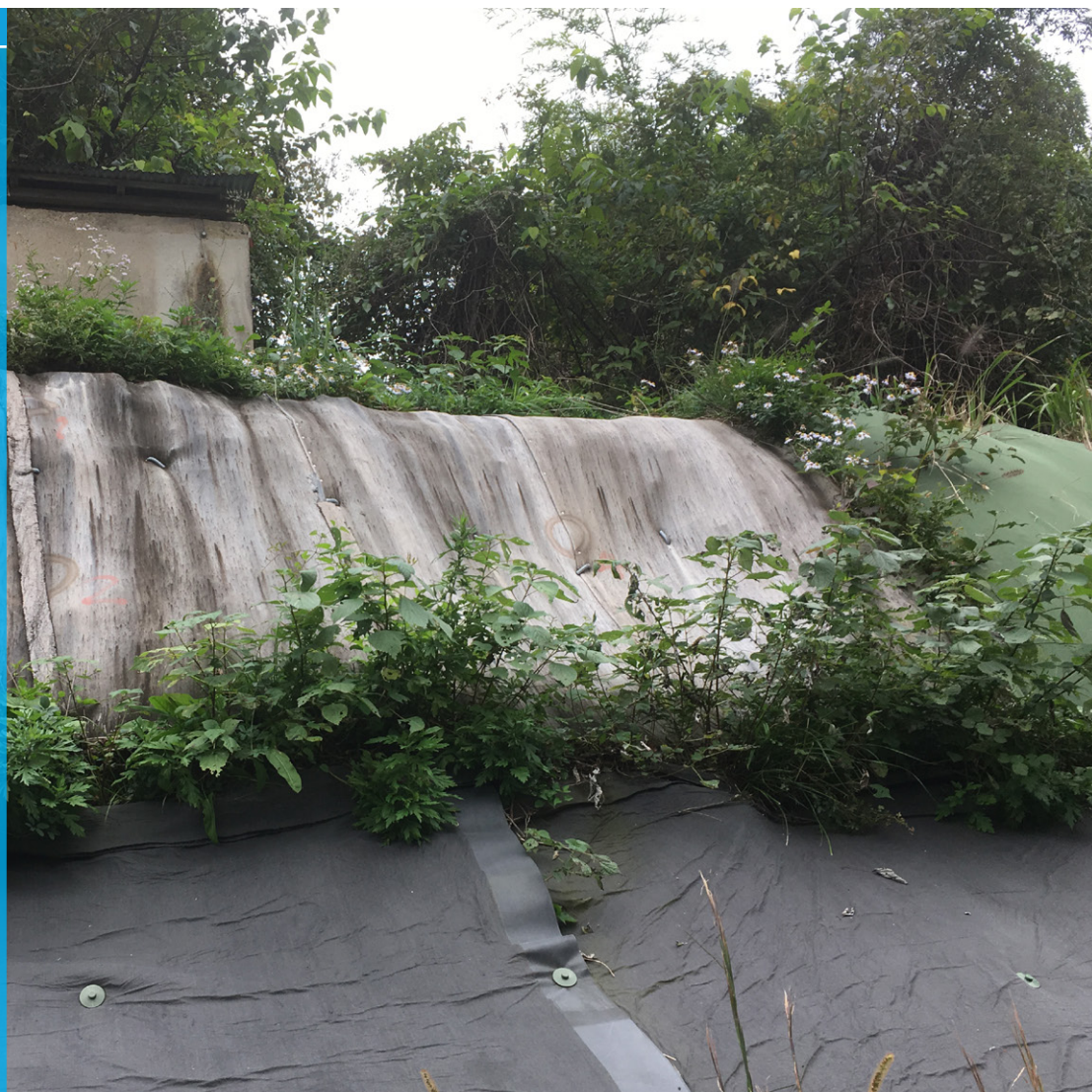
Trial CC section 26 months after installation
