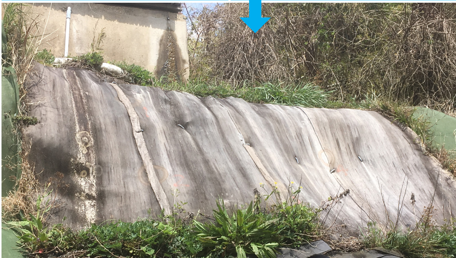
Day 816 - CC is beginning to moss over with age and still shows no signs of weed protrusion
