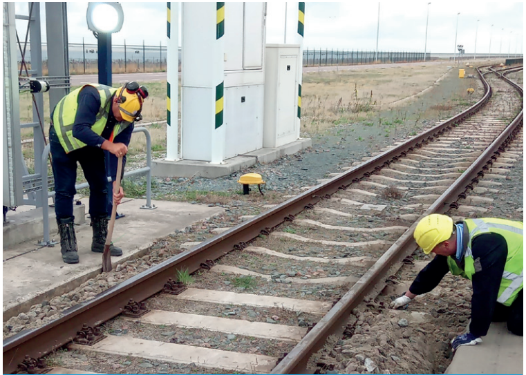
Removal of stones and rocks from trackside prior to install
