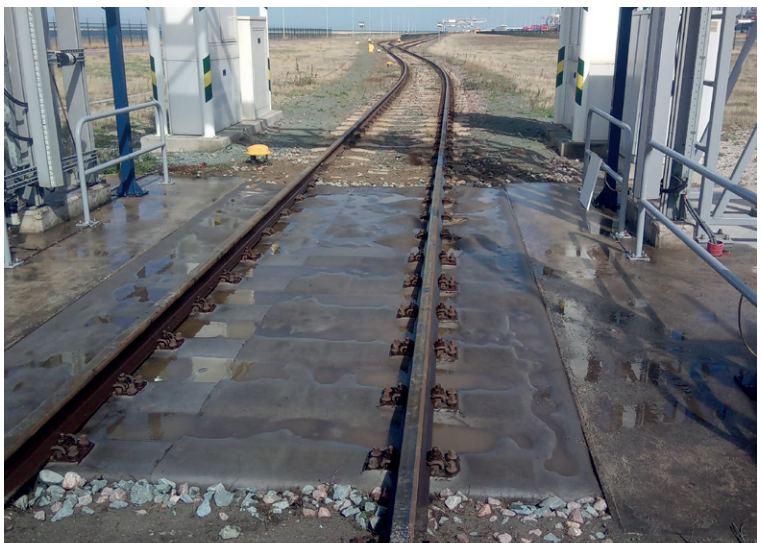
Completed section following hydration
