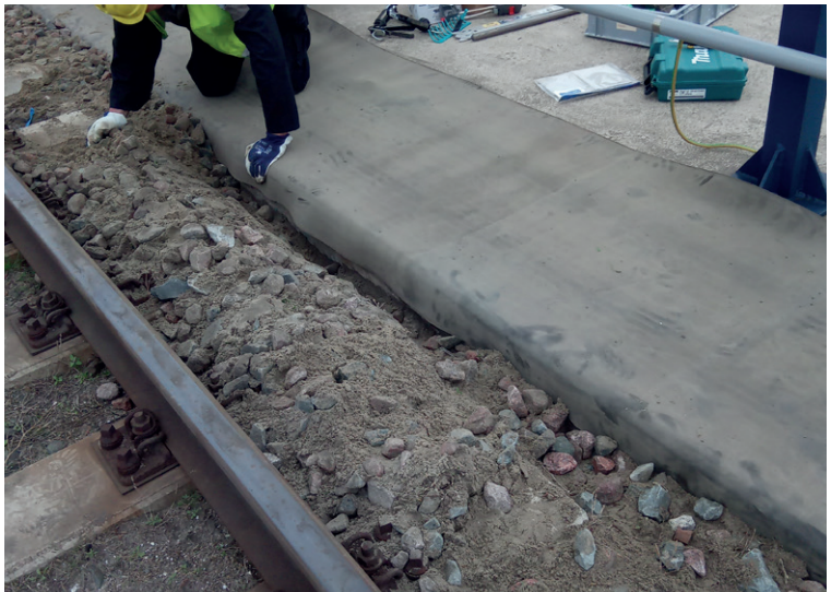
Edge of CC buried in anchor trench and covered with stones and small rocks
