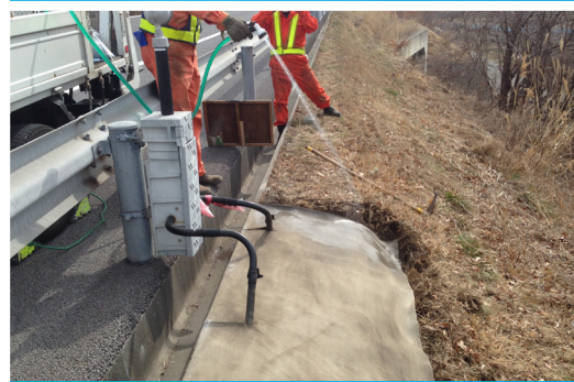
The CC was secured then hydrated
