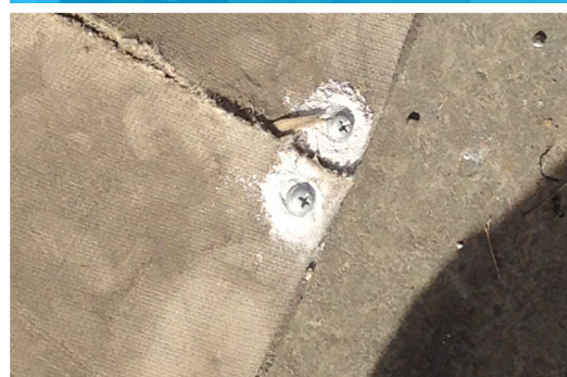
Screws were inserted through the CC and concrete
