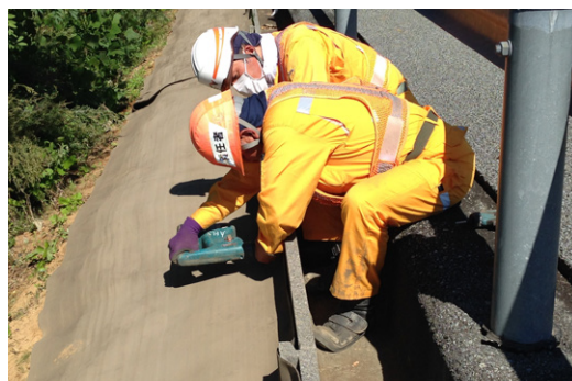
Fixing the CC to concrete infrastructure using screws
