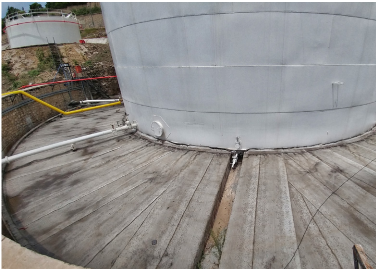
Completed bund floor area installation
