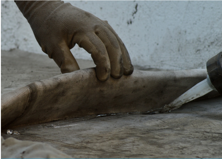
Adhesive sealant used to joint overlaps and prevent ingress
