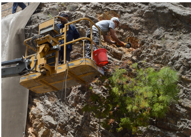
Removal of tree from slope prior to installation
