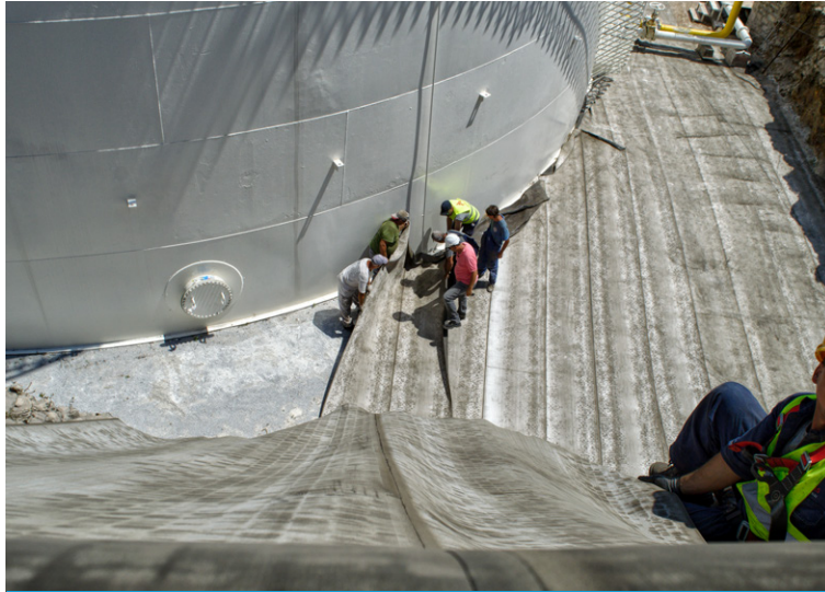
Length of CC deployed down slope and along bund floor
