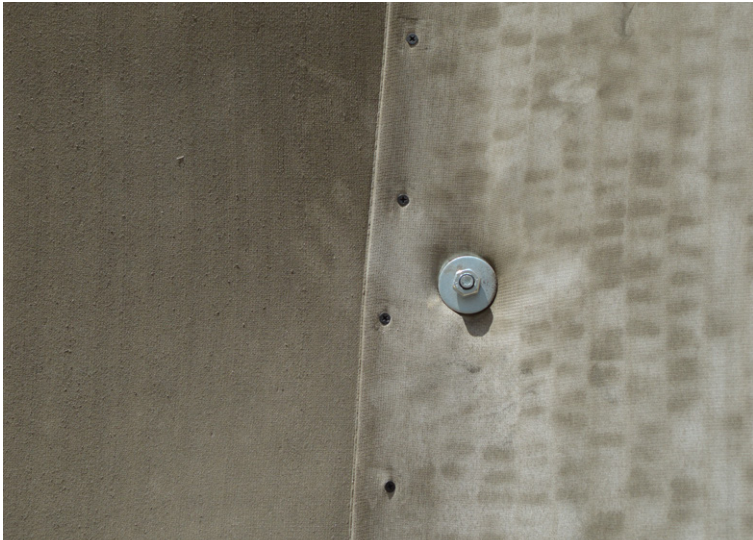
Screws and Hilti nails used to joint and fix CC to slope
