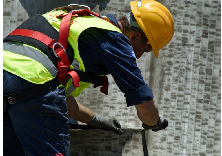
Cutting CC to required length to prevent wastage
