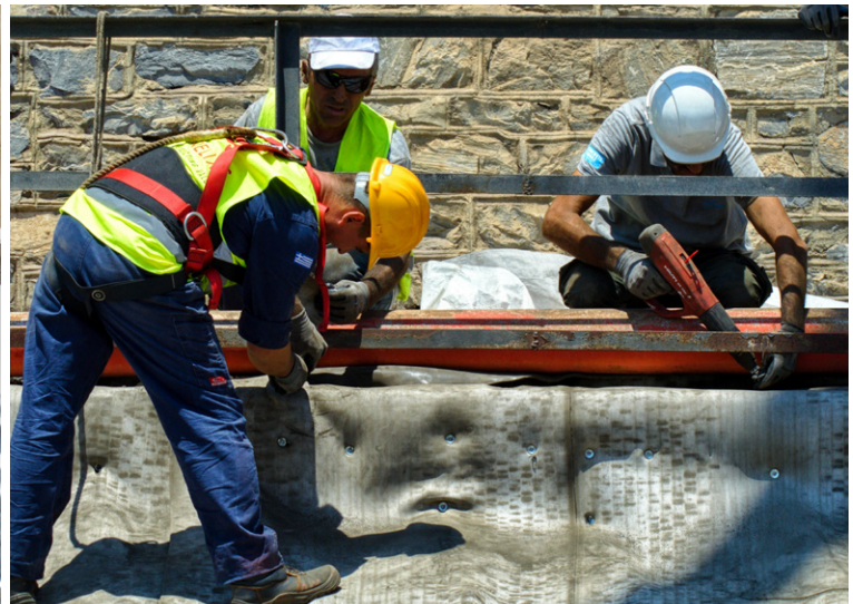
Fixing of CC to concrete wall at slope crest using Hilti nails
