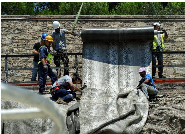
CC 2-wide rolls deployed from spreader beam from slope crest
