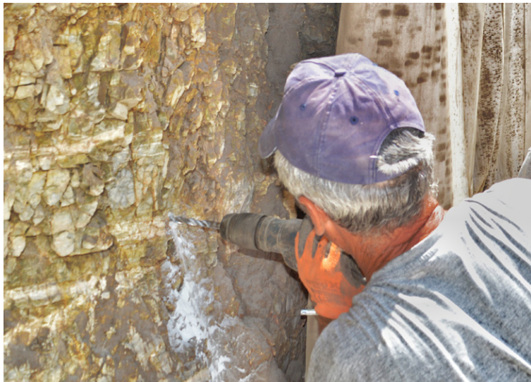
Drilling into rockface to allow fixing of CC to slope
