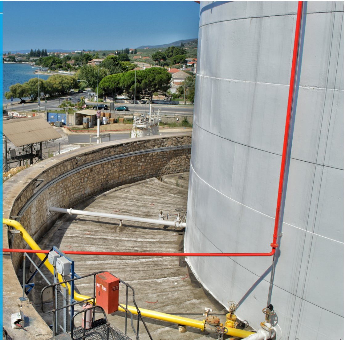
Completed CC lined bund area floor
