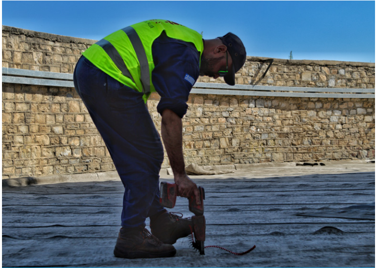
Overlaps on bund floor jointed using screws
