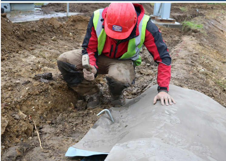
Fixing into the anchor trench
