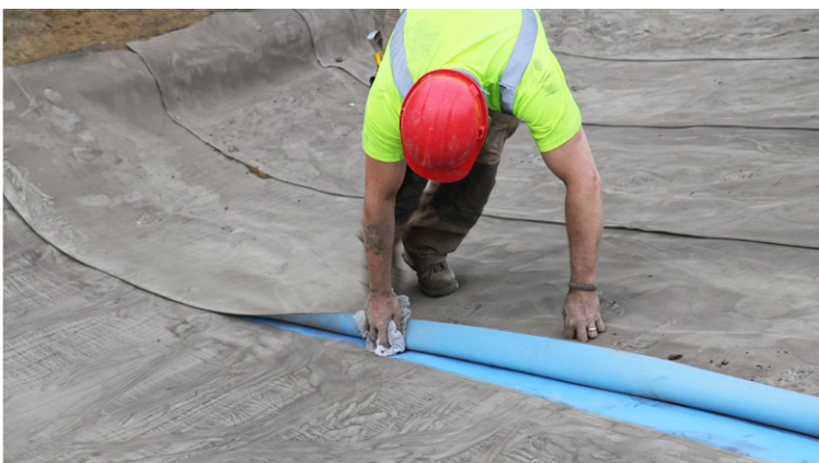
Cleaning the geomembrane faces to be welded
