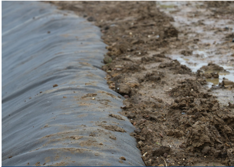
Backfilled anchor trench
