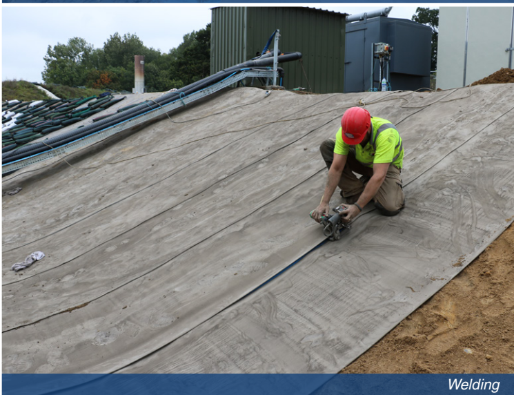
Fixing into the anchor trench
