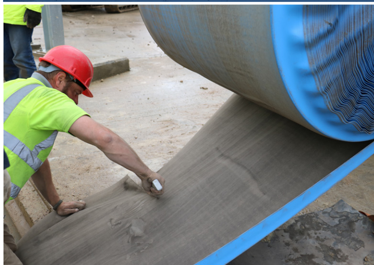
Cutting the CC Hydro™ to length
