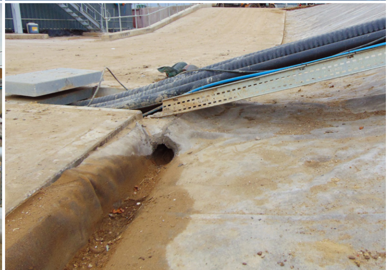
Toe drain details
