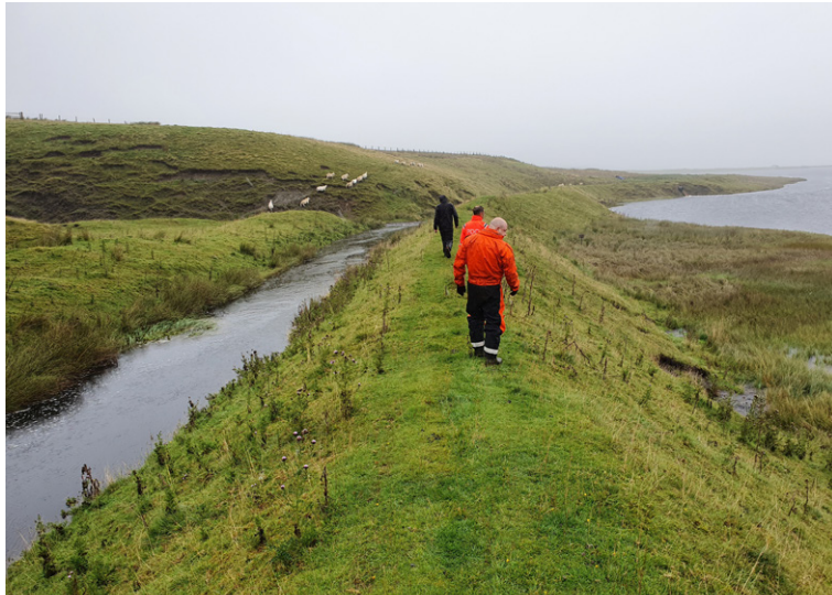
Leakage at the downstream toe of by-wash embankment
