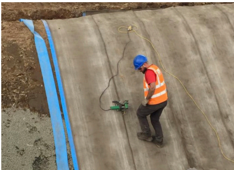
Thermal welding of CCH overlaps
