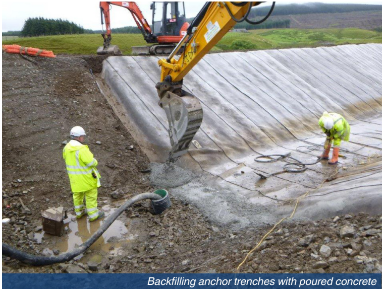
Facing upstream prior to poured concrete backfill
