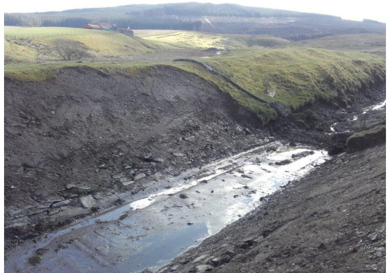
Draining & excavation of by-wash channel
