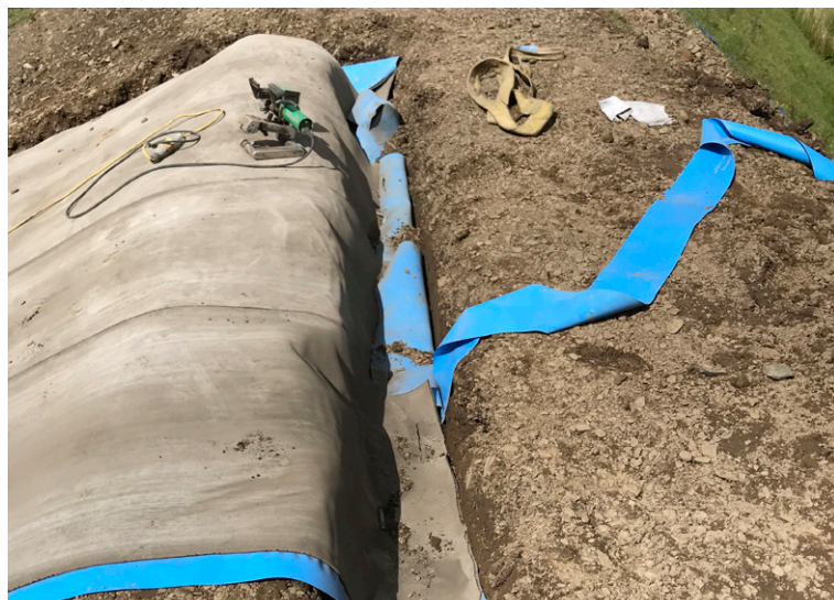
CCH terminated into 150mm anchor trenches prior to backfill
