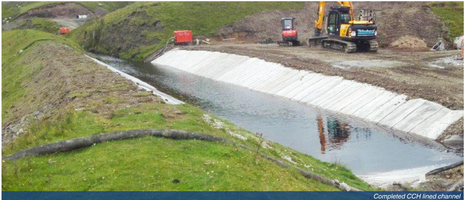
Completed CCH lined channel
