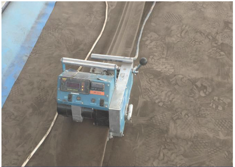
Mechanical thermal welding
