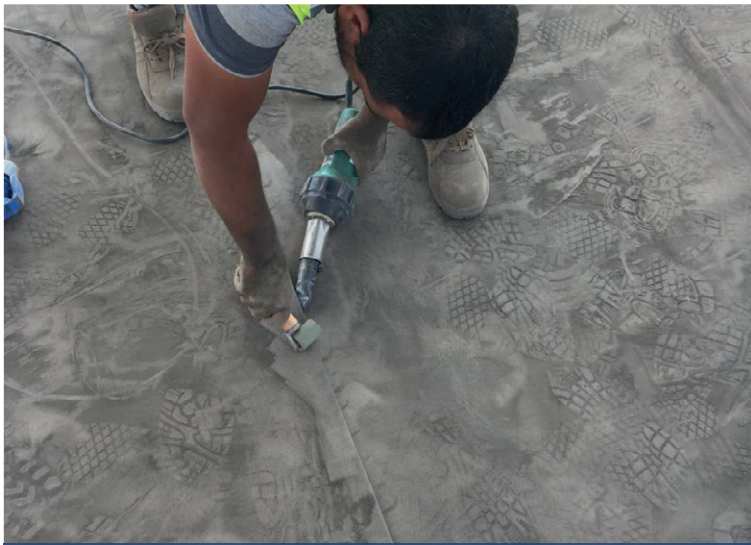
Thermal welding using hot air gun and roller
