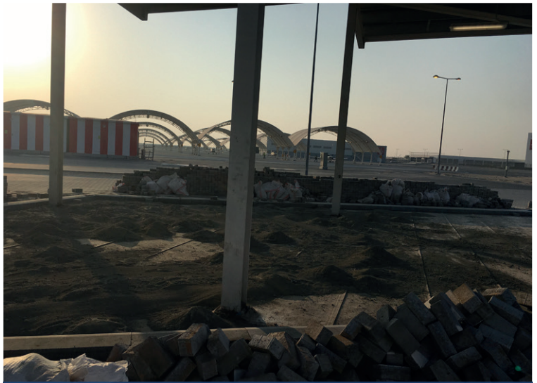
Covering completed CCH installation with sand prior to paving
