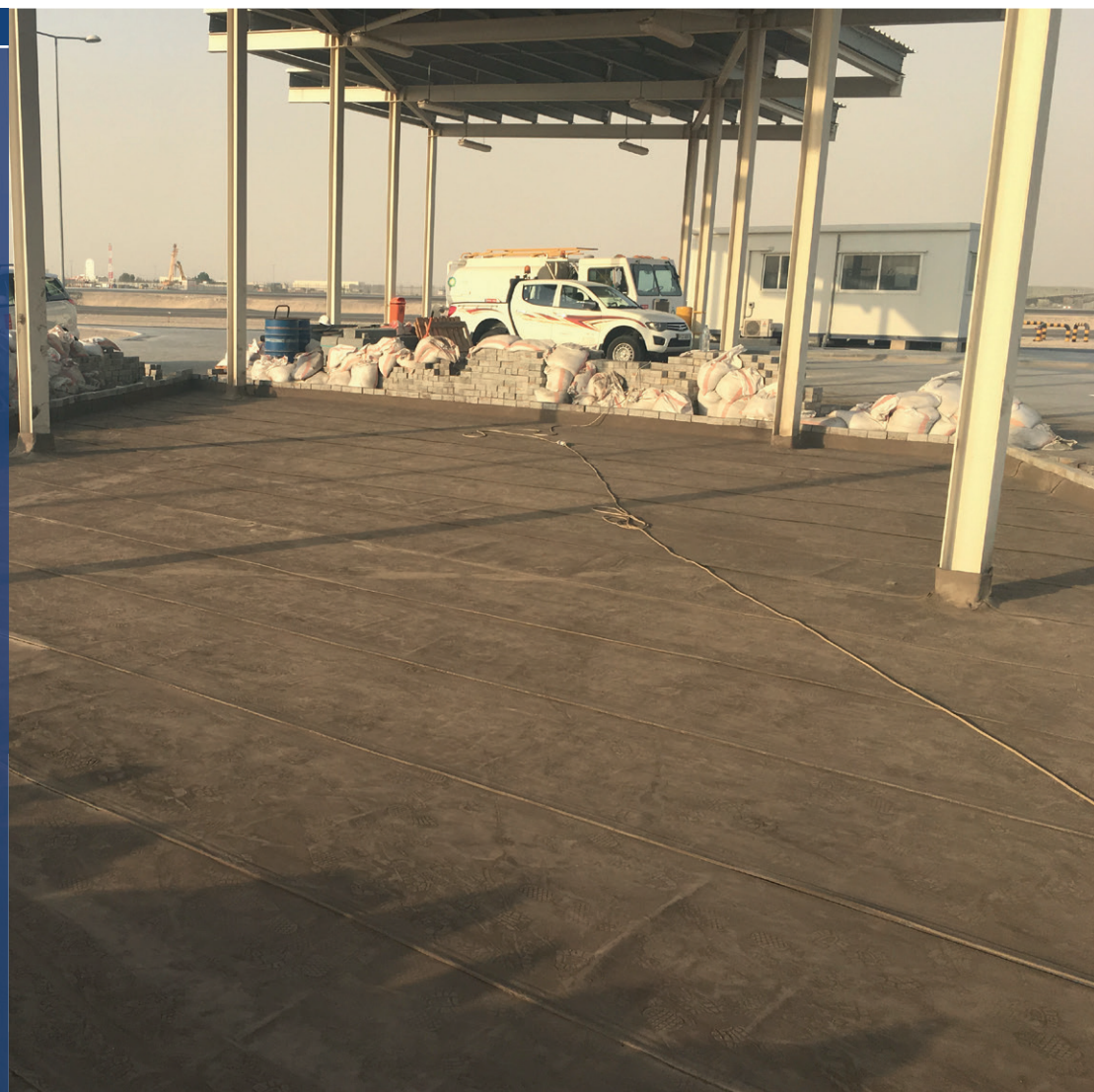
Completed CCH installation prior hydration and paving
