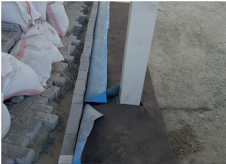
Laying first length of CCH and cutting to accomodate posts
