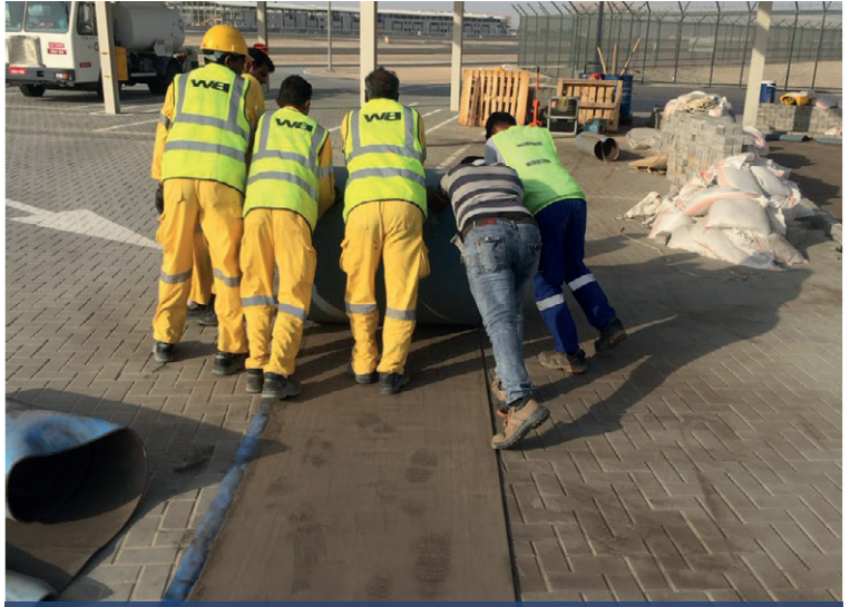
Unrolling CCH to cut material to required length prior to works
