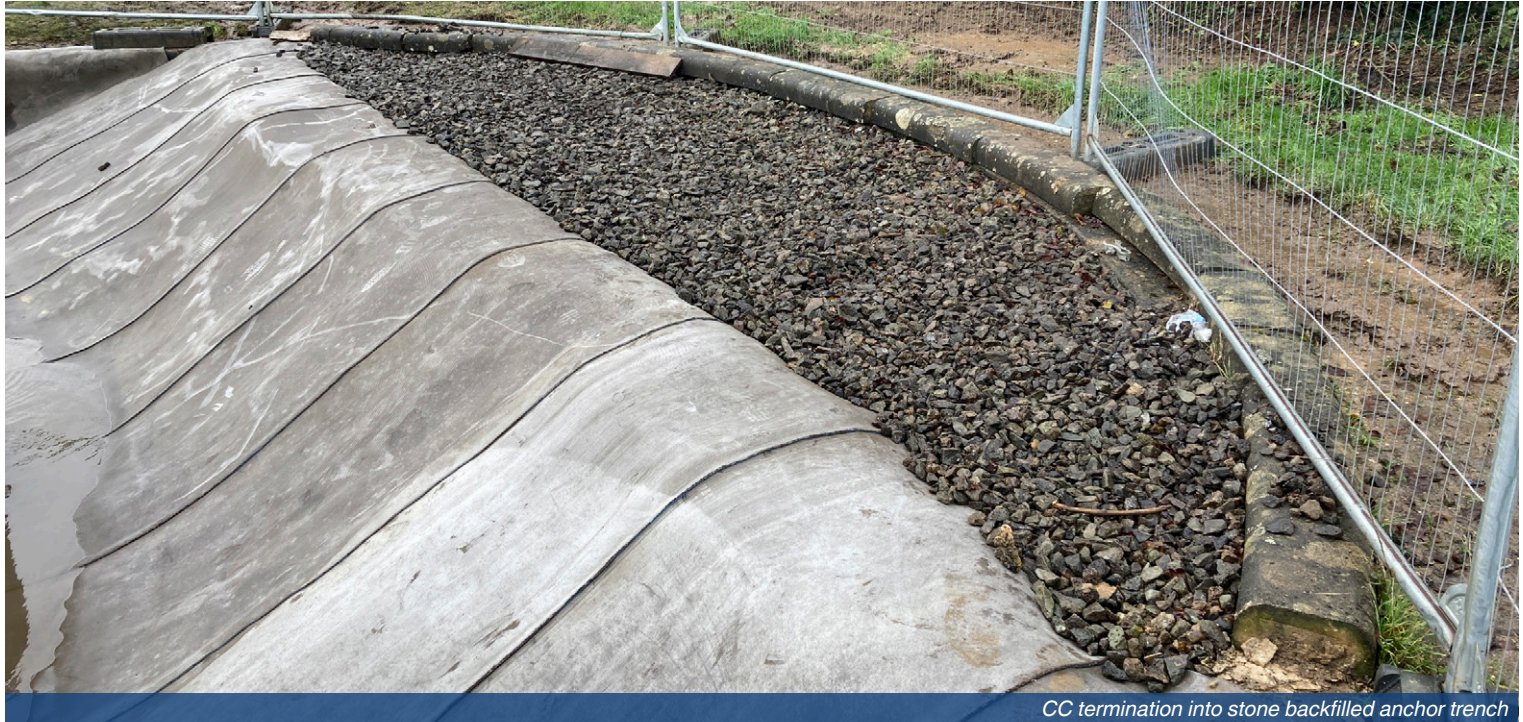
CC termination into stone backfilled anchor trench
