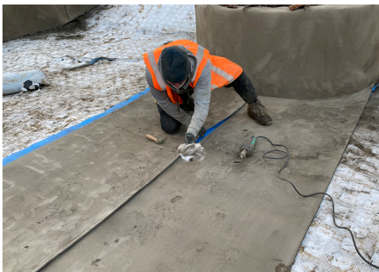
Thermal welding of CCH lengths along tank floor
