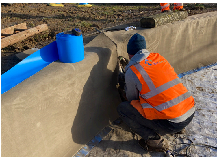
Thermal welding of the CCH around the tank wall
