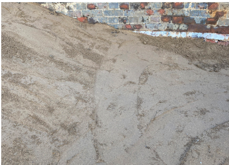
Sloped section of tank created with stone and sand
