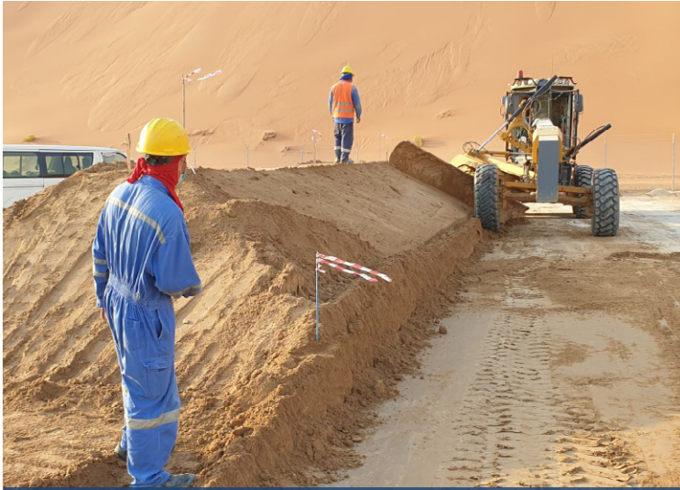
Construction of dykes
