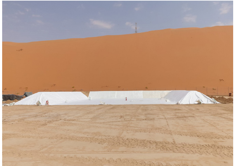
Geotextile laid to act as additional barrier between substrate and CC Hydro™
