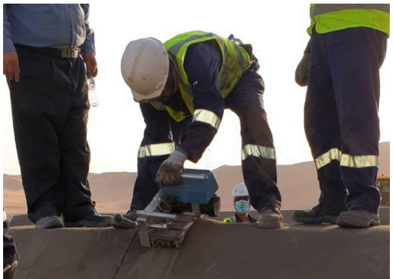
CC Hydro™ lengths thermally welded for impermeable joints
