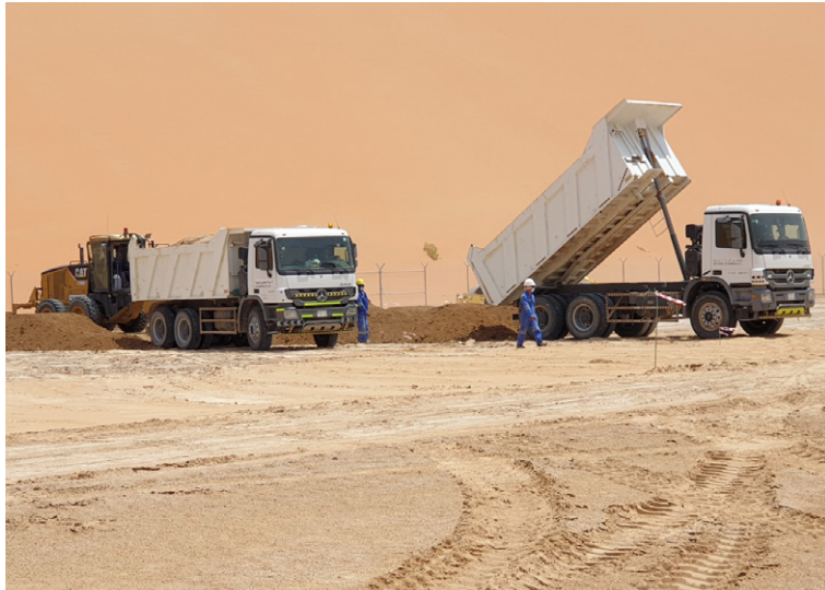
Delivery of first marl layer for area base
