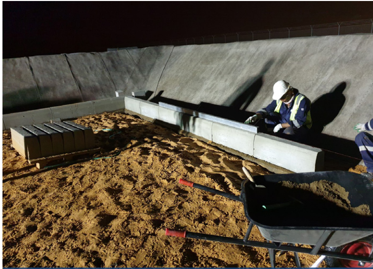
Sand layer installed & curb stones placed around base perimeter
