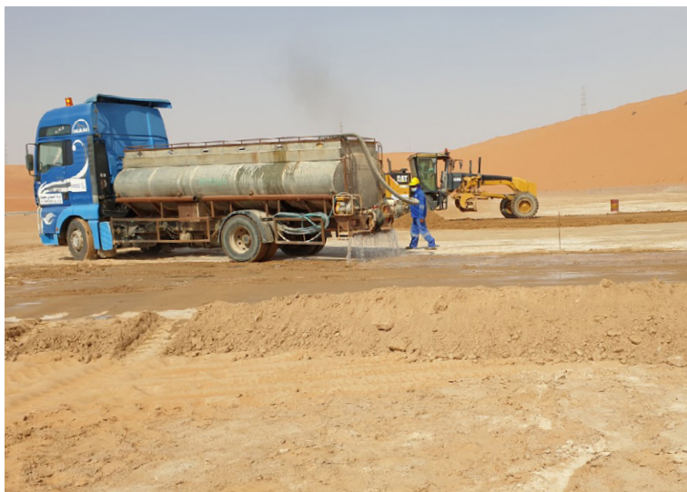
Hydration of marl following compaction
