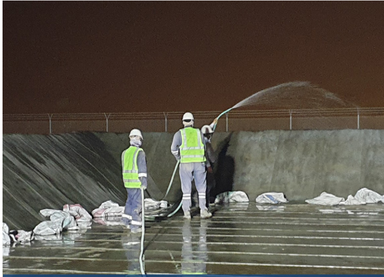
First hydration given at night to prevent evaporation
