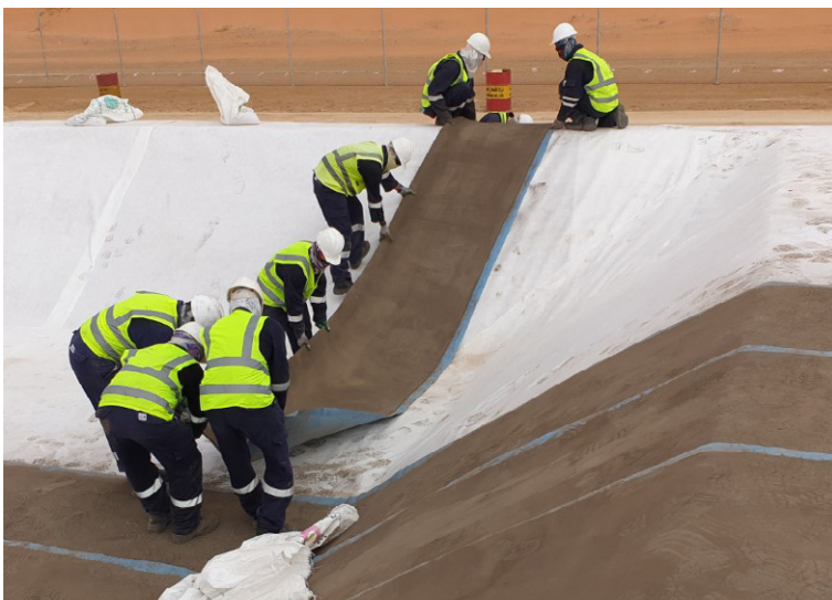
CC Hydro™ laid transversely across treatment area & vertically down dyke wall
