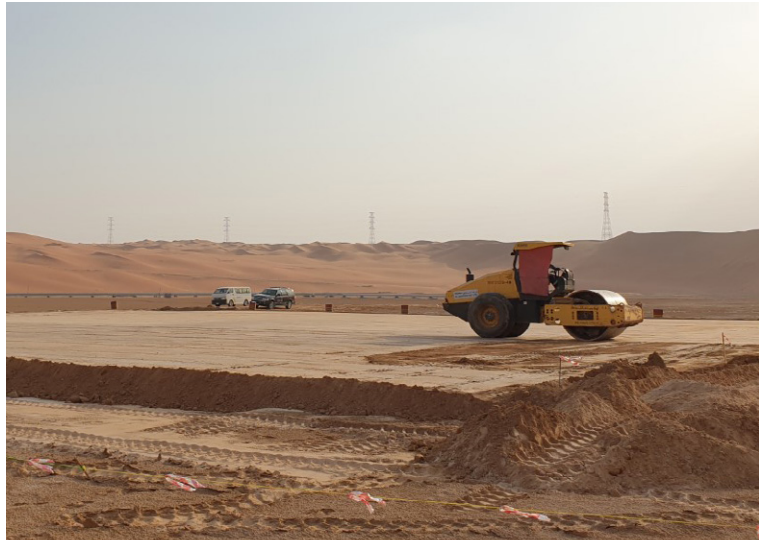
Compaction of marl layers
