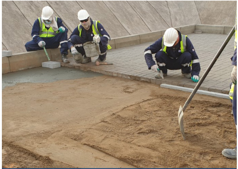
Interlocking paving installed over the base to create traffickable surface
