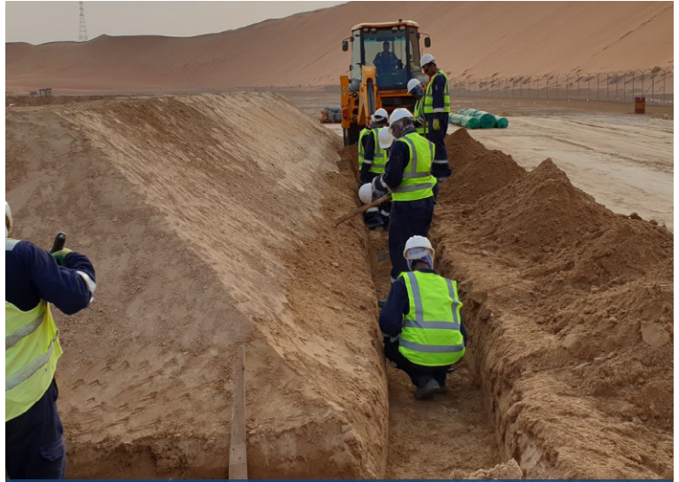
Creation of anchor trenches behind dyke walls
