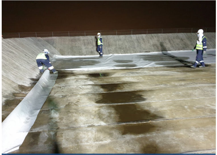
Second geotextile layer placed over hydrated CC Hydro™ base
