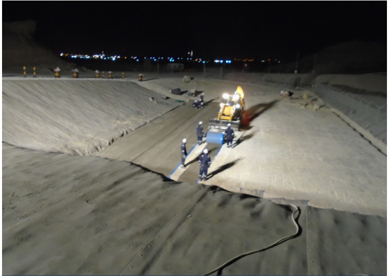
Deployment of CCH on ground below slopes
