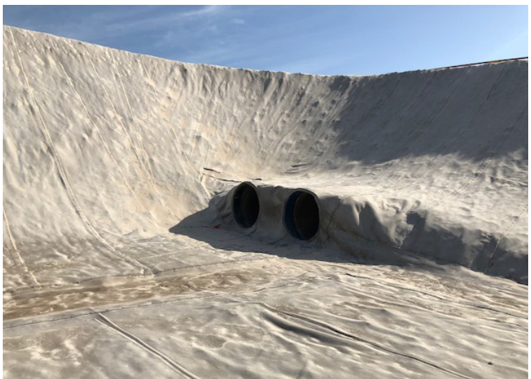
CCH installed around outflow pipes
