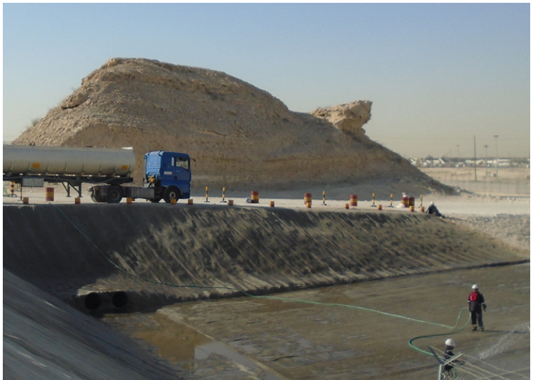
Hydration of CCH was carried out twice with 2 hour interval
