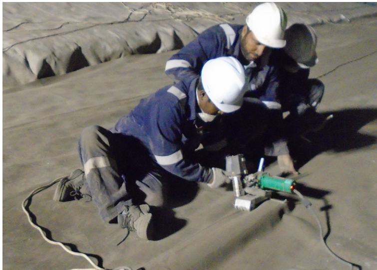
Thermal welding of CCH layers for impermeable joints
