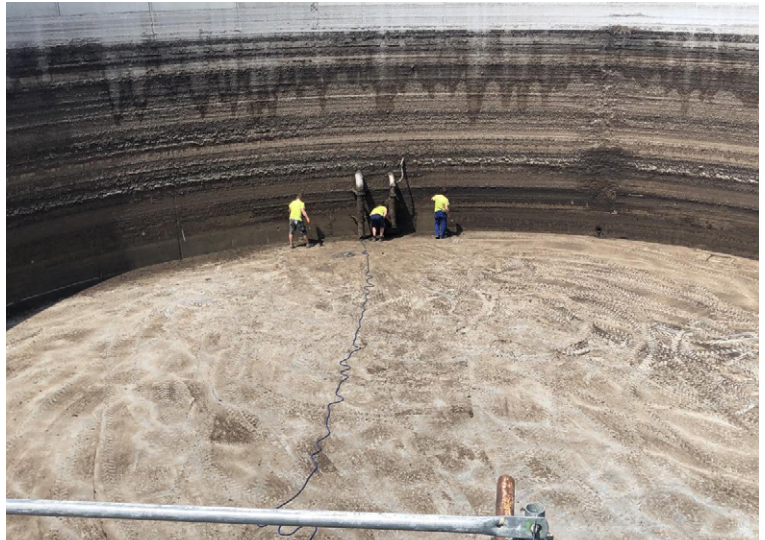
Clearing digestate from walls following emptying of tank
