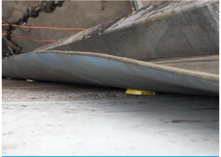
CCH was welded to Sika WP discs to ensure flush contact with the wall
