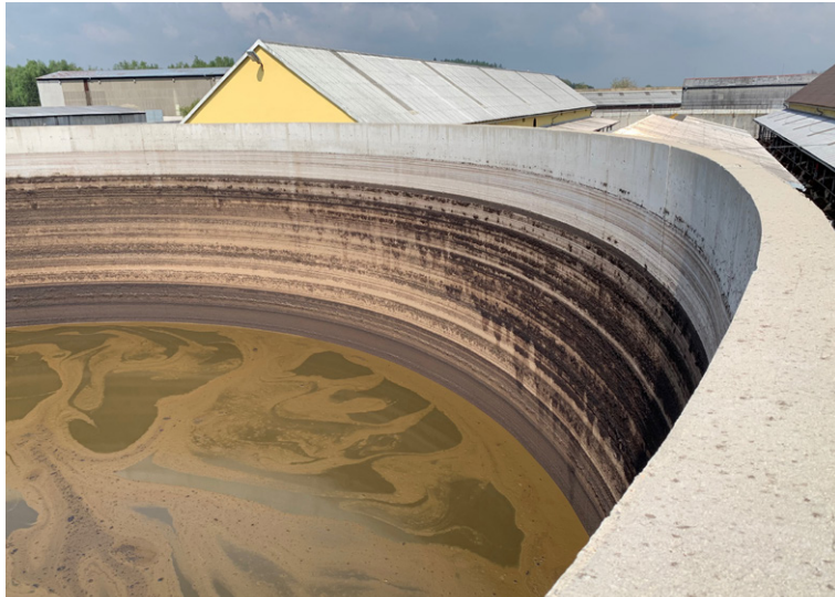
The digestate tank measured 9m high and had 300mm thick walls
