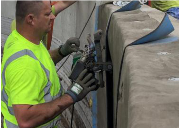
Lengths of CCH were welded together using a Leister Twinnys S
