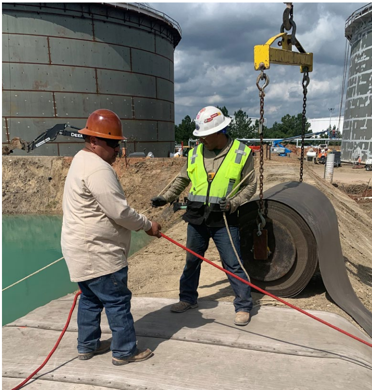
CC5™ installed with a spreader bar
