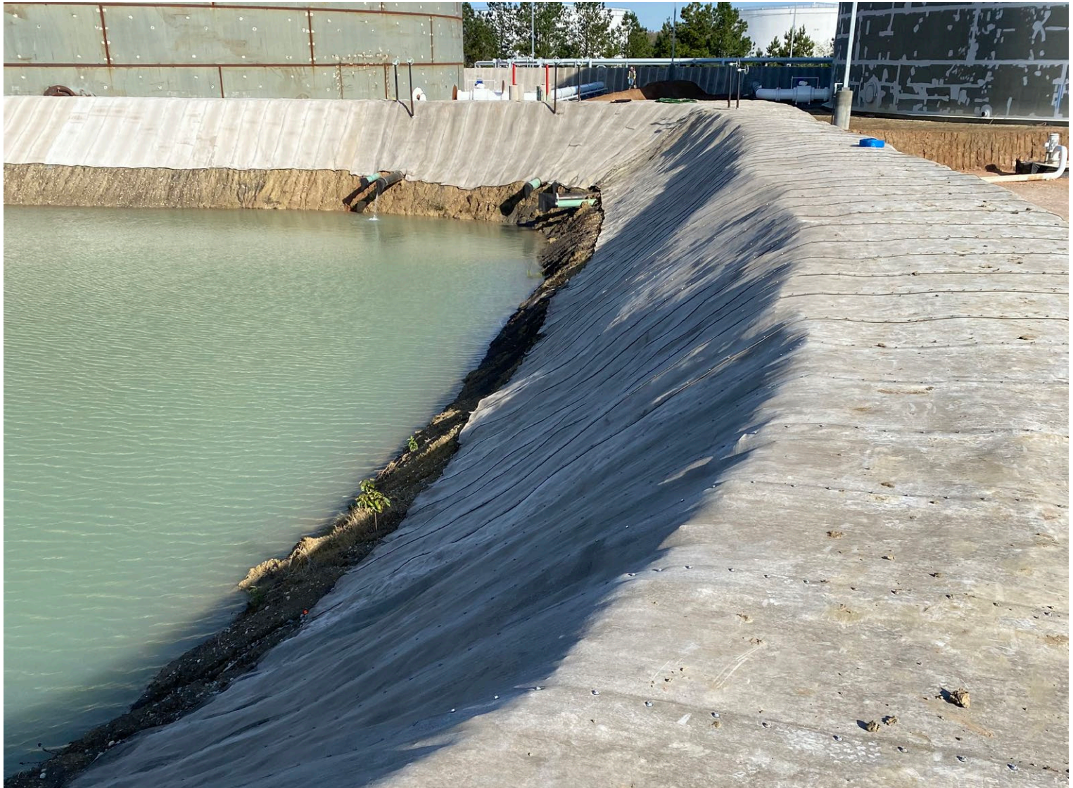
Completed slope protection works with overlaps secured with 1.25 inch screws
