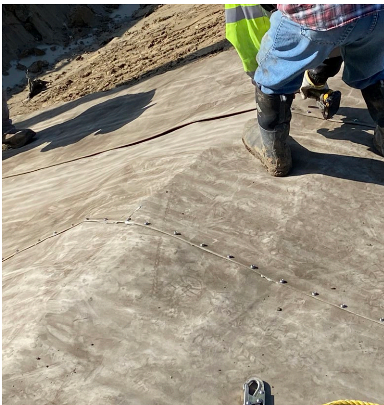
Overlaps secured with 1.25-inch self-driving stainless steel screws
