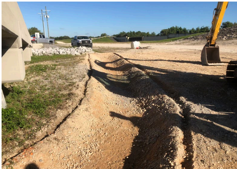
Ditch re-profiled using excavator
