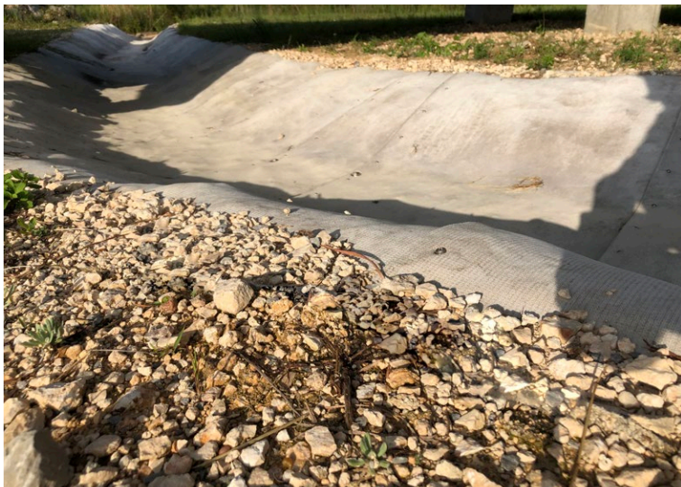
Backfilled anchor trenches
