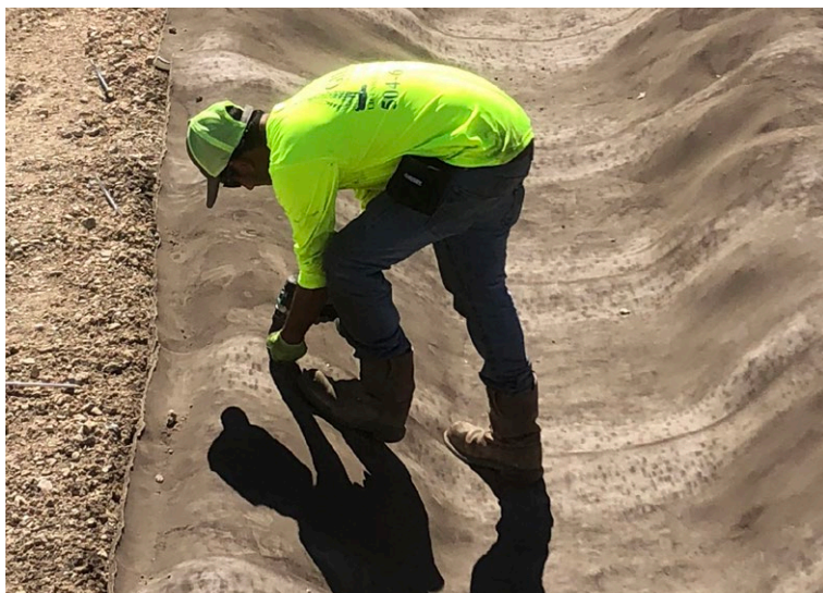
Overlaps secured with stainless steel screws
