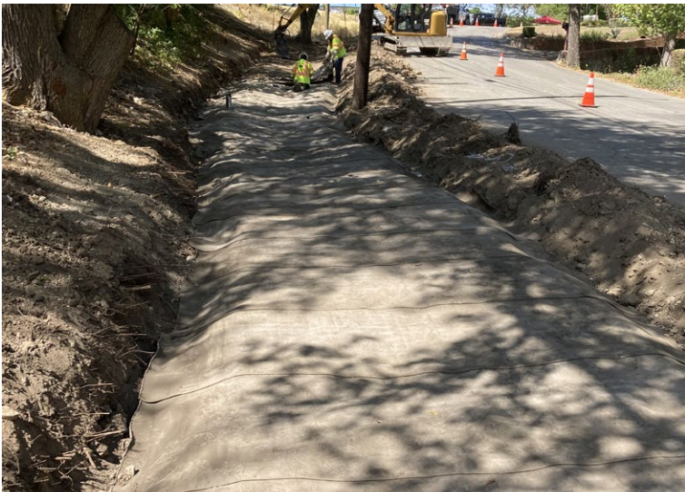
CC5™ Laid transversely across the ditch
