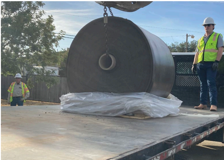
Bulk Roll of CC5™ lifted using excavator and spreader beam
