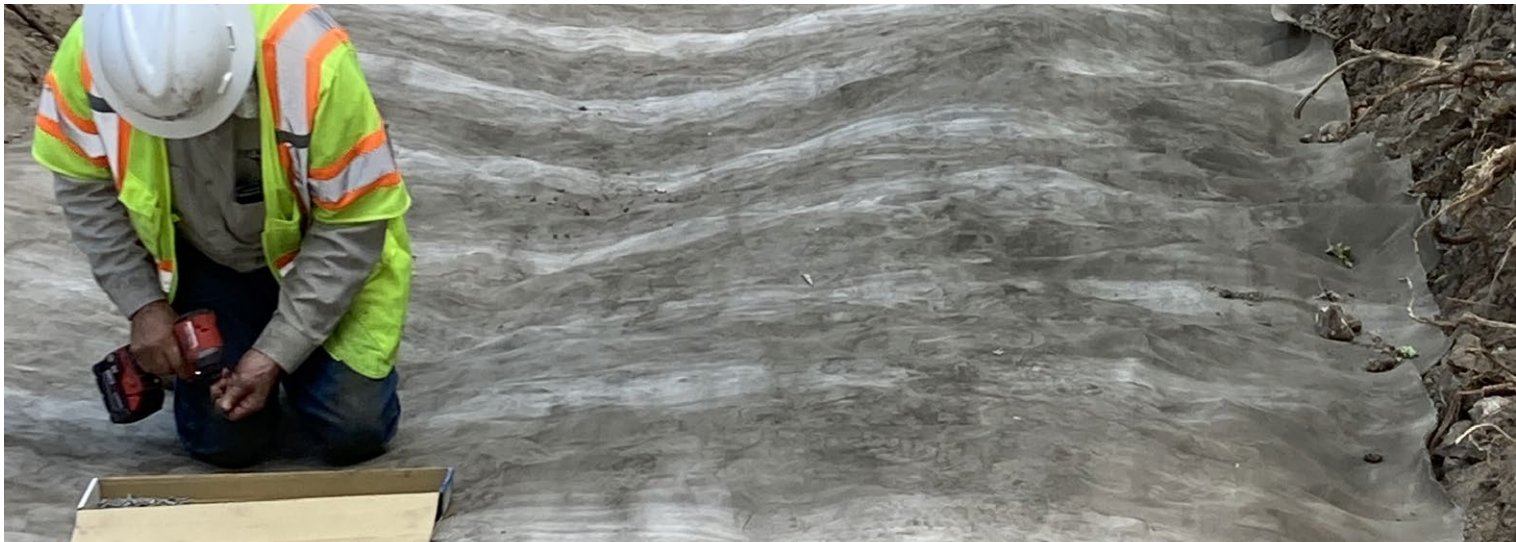
Overlapped layers secured with stainless steel screws
