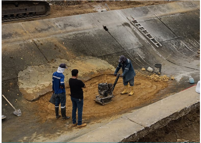
Damaged concrete infilled with compacted earth
