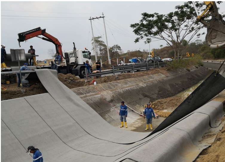
CCX-M™ deployed from flat bed truck and pulled across with an excavator
