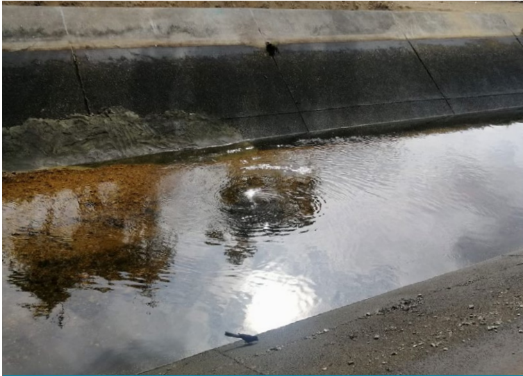
Water loss from hole in canal
