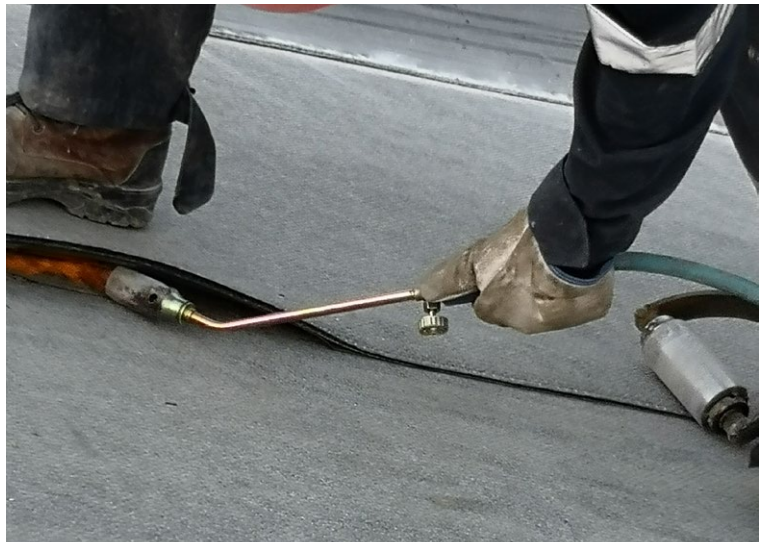
CCX-M™ thermally bonded using propane gas torch
