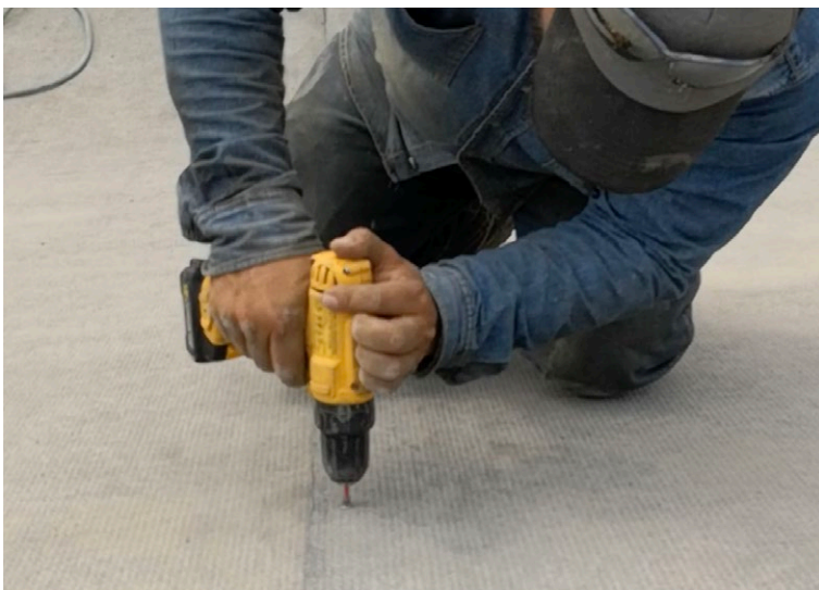
CCX-M™ secured with short length stainless steel screws
