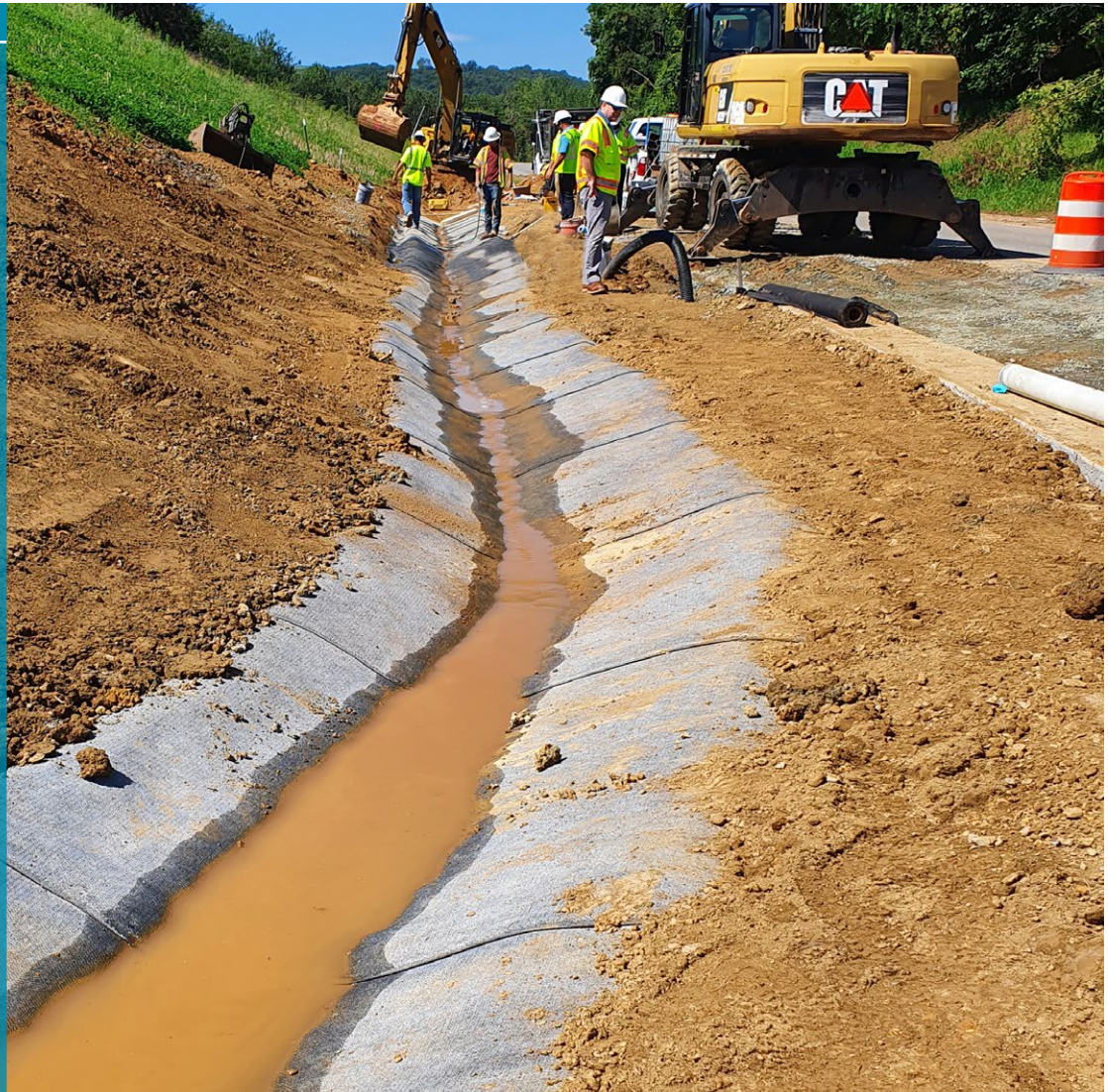
Completed CCX-M™ Installation
