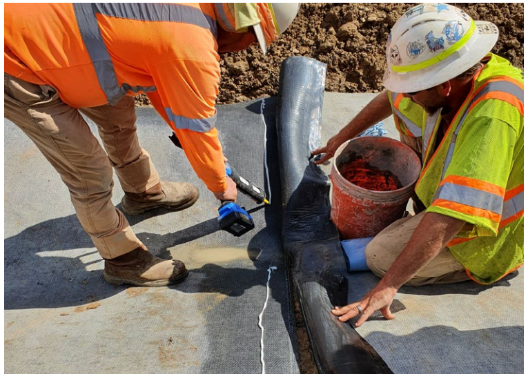
Overlapping layers sealed and screwed
