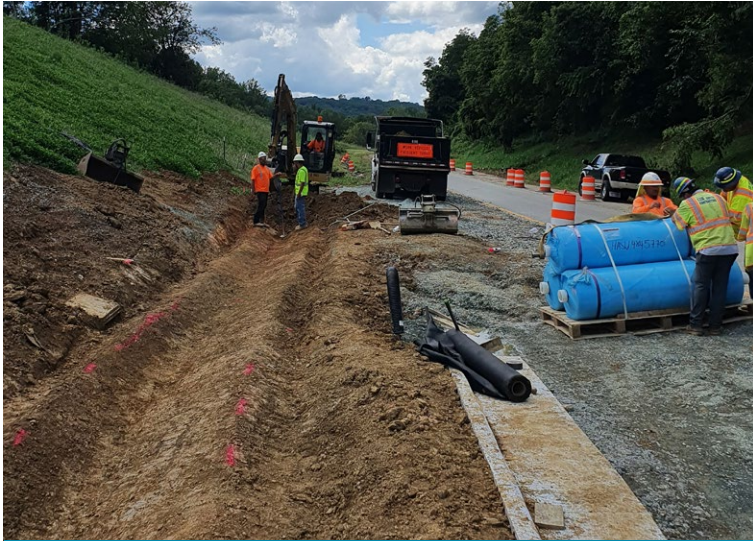
V-ditch dug with excavator
