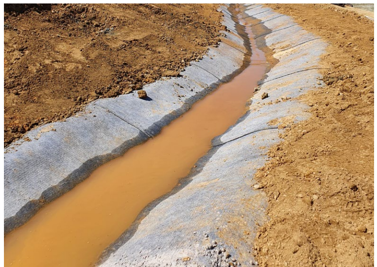
Anchor trenches back filled
