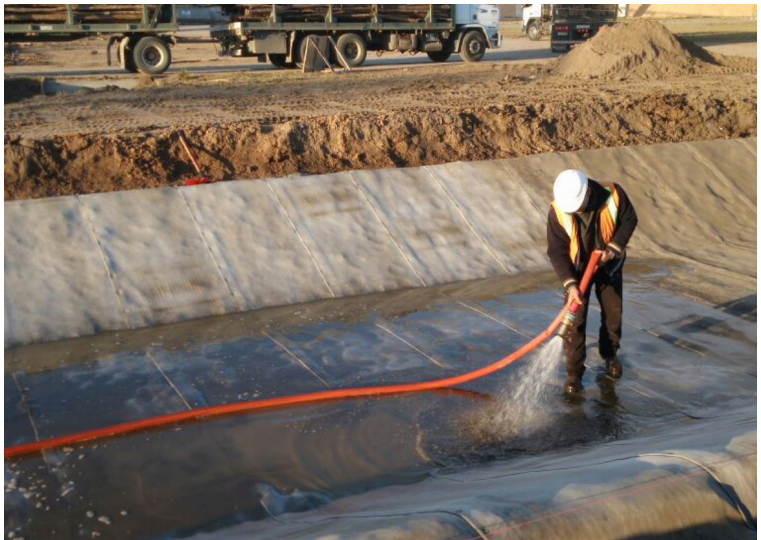
The CC was hydrated following completion of installation
