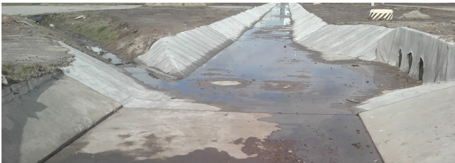
A section of the channel including a headwall, meeting concrete infrastructure and a junction
