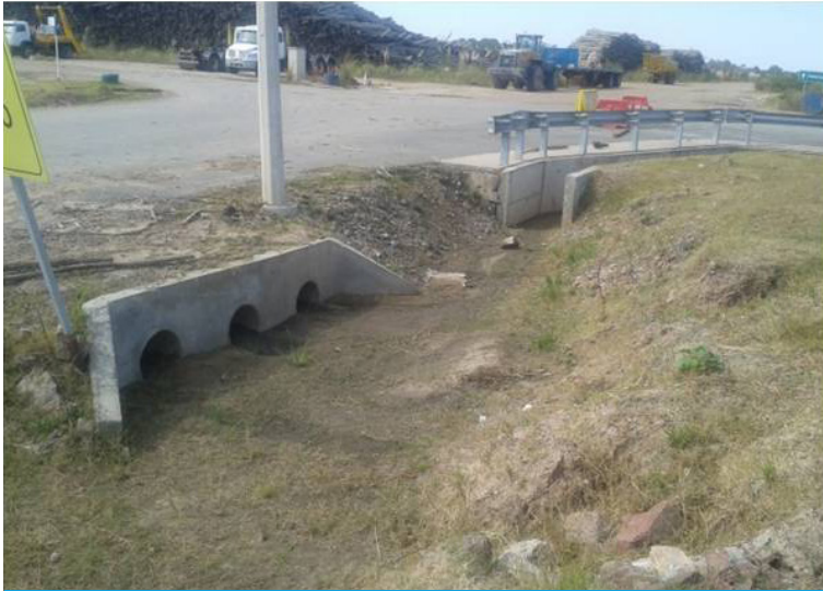
The area was graded, levelled and rid of vegetation prior to installation
