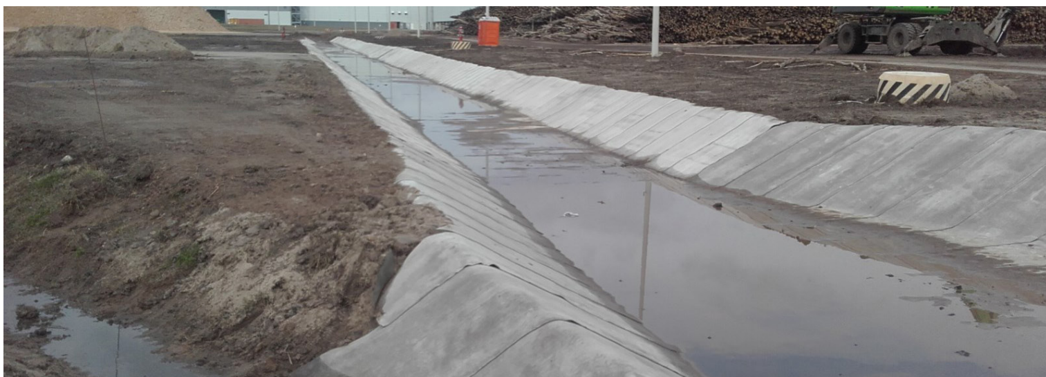
The termination of the CC at the junction
